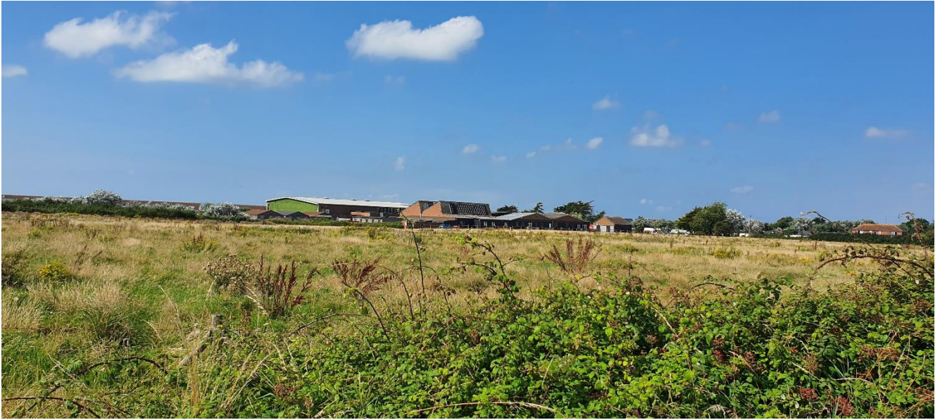
Fig. 7: View towards the existing Medmerry Hub from the proposed back of house facilities cluster.
