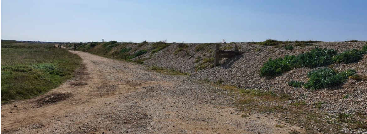
Fig. 56: View Across Southern Flood Defence
