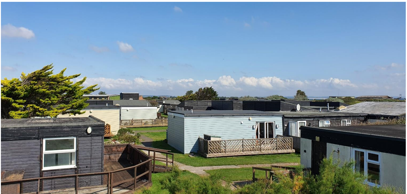
Fig. 6: View of existing accommodation and landscaping seen throughout the site location – accommodation is seen to be in a poor condition with many units off sale to the public.
