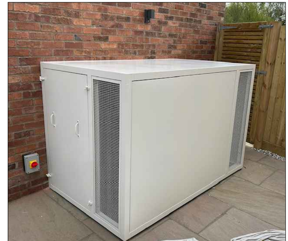
Photo of Acoustic Enclosure
