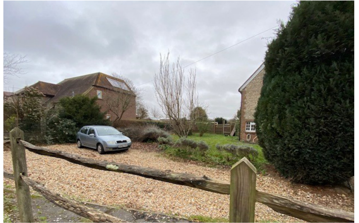
6 View of existing parking court to no. 27
