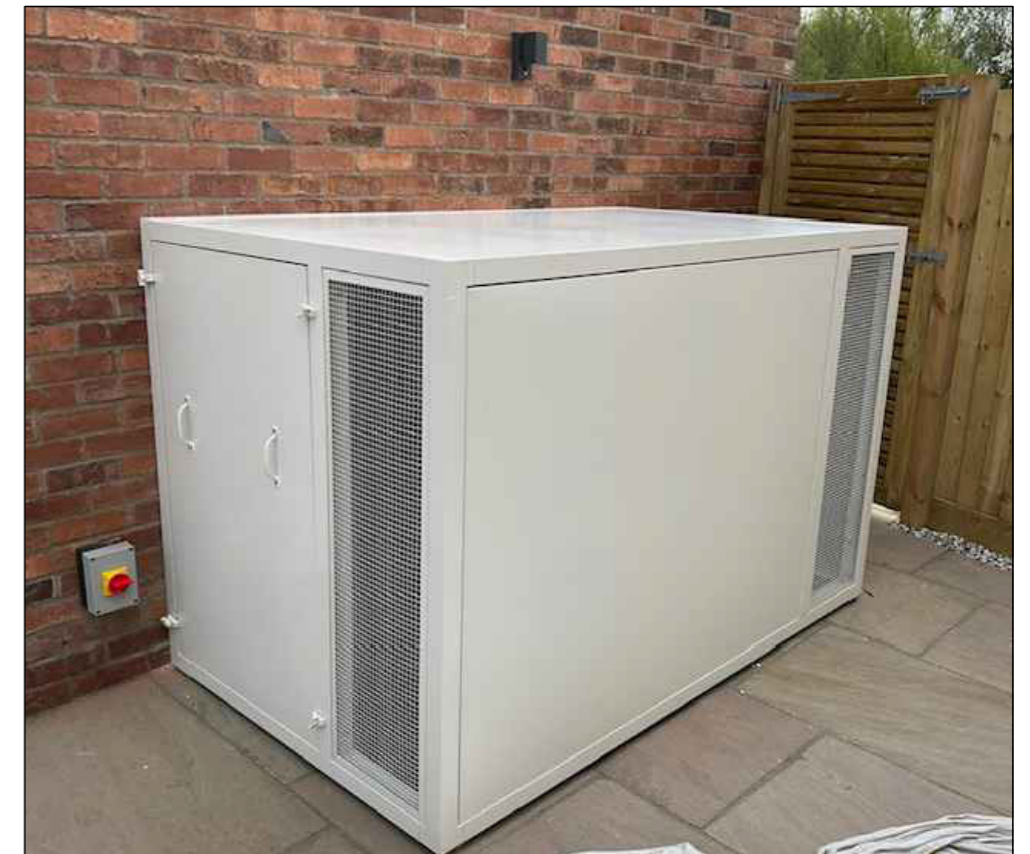
Photo of Acoustic Enclosure
