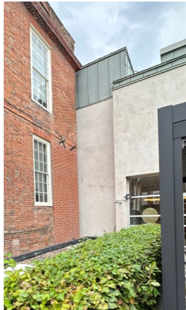
4. Pallant House Gallery in Chichester. Stone coloured render used in historic context
