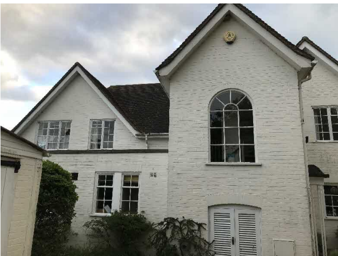
Photo 4. Building viewed from E.
