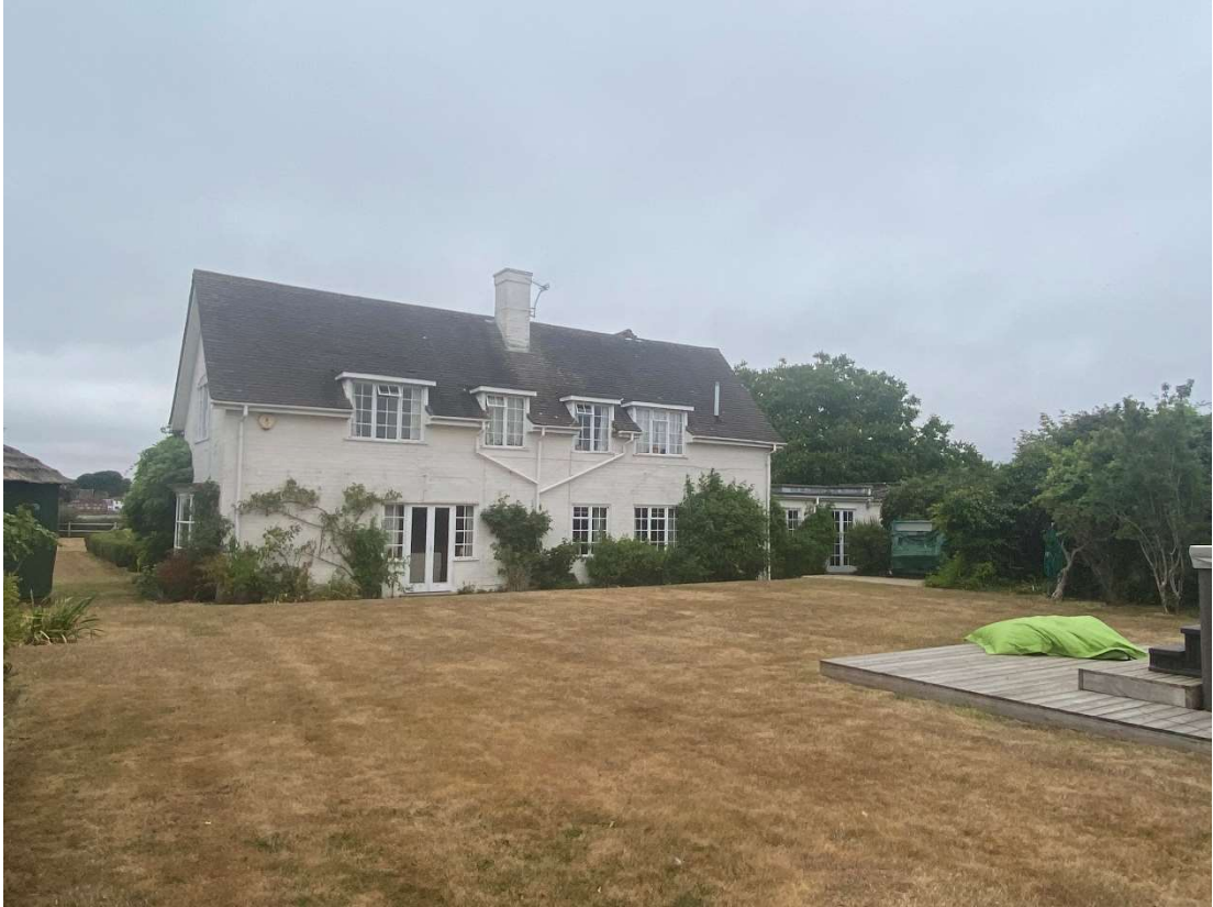
Photograph 7: View of the house rear elevation.
