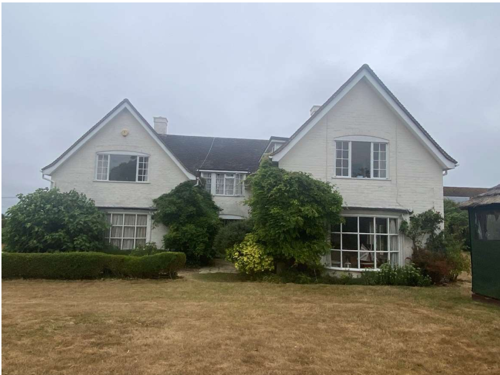
Photograph 6: View of the house- western side elevation.
