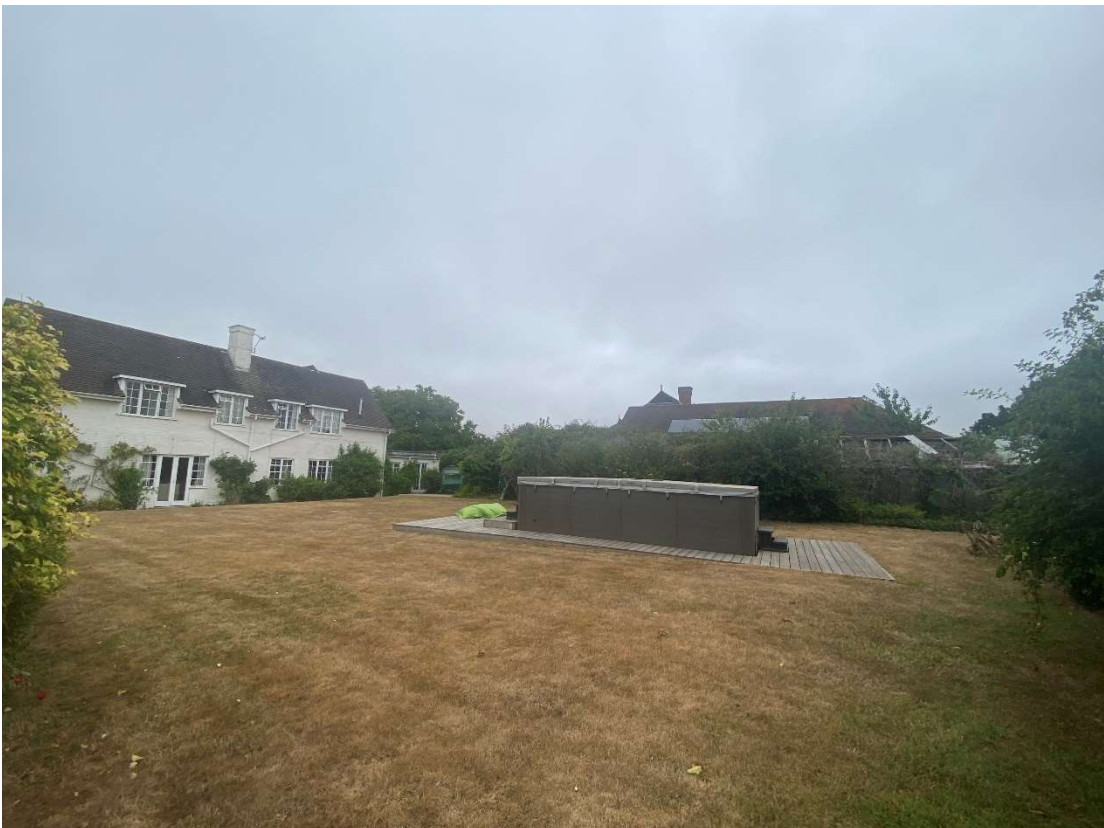
Photograph 8: View of the house rear elevation, rear garden area and glasshouse.
