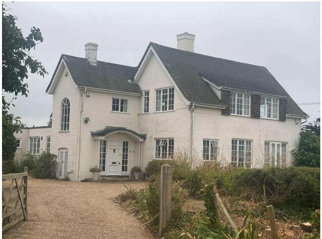
Photograph 4: View of the house from the top of the access drive.
