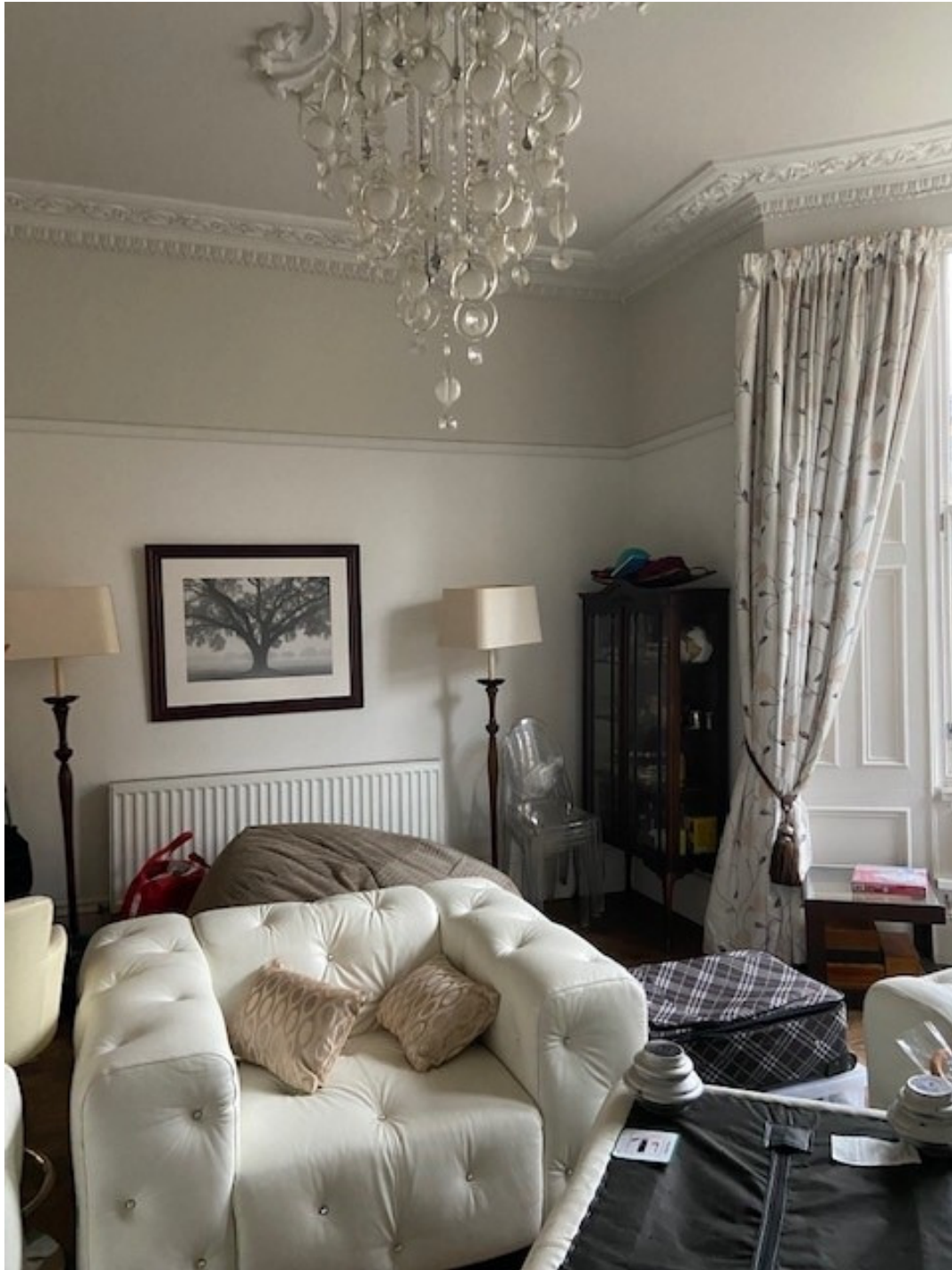
Existing lounge and cornicing reinstated following removal of bathroom conversion.
