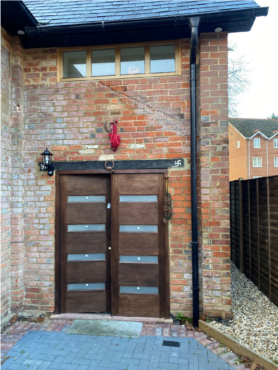
Existing Front Doors
