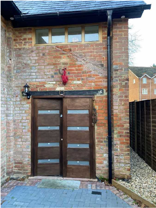
Existing Front Doors
