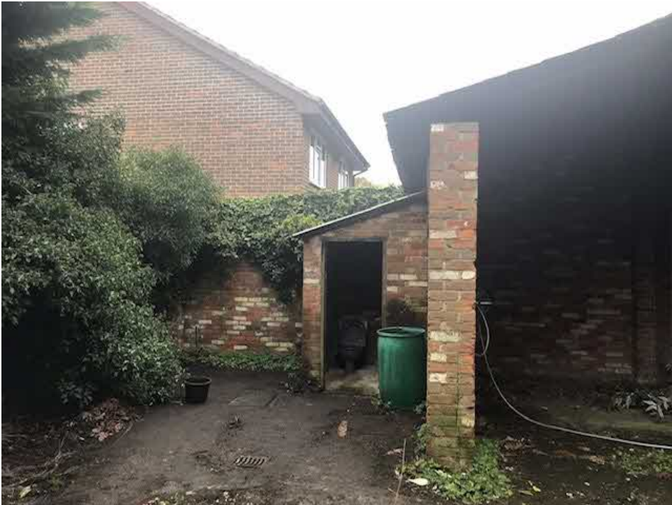
North Wall (Original Building) © Client
