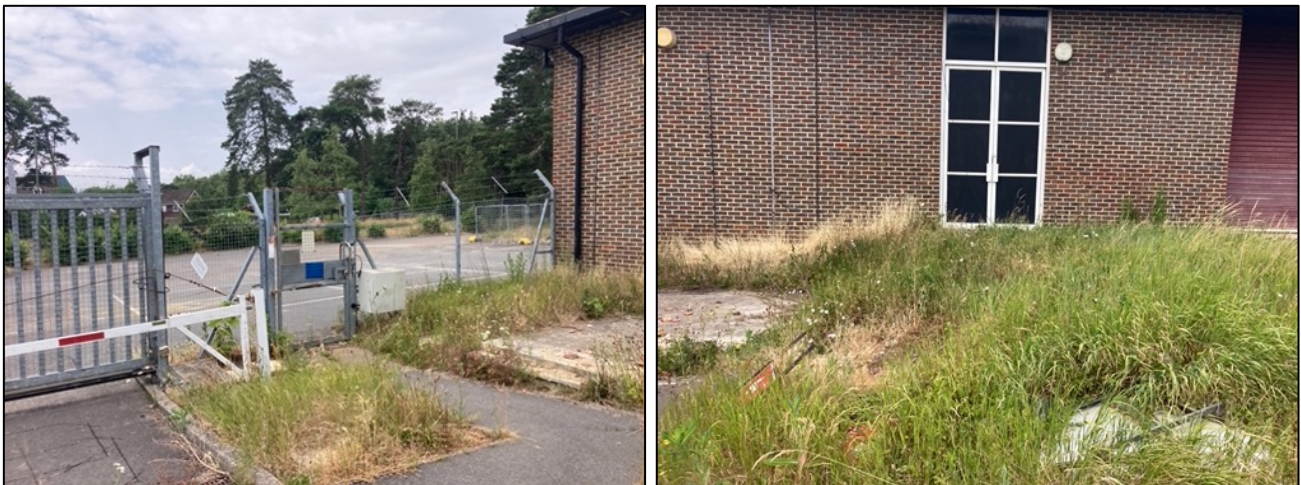
Photograph 1a (left) & b (right). Left – View north-east over the car park and barbed wire fencing. Right – Area of grassland along the southern elevation of the museum building.
