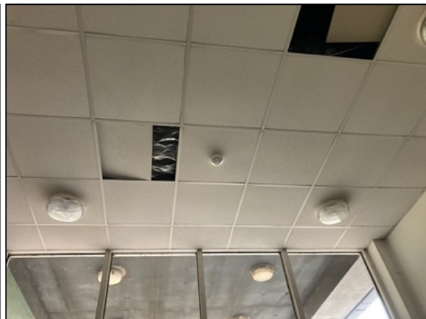
Photograph 14a (left) & b (right). Views of slipped ceiling tiles in the suspended ceiling over the side rooms.
