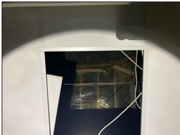
Photograph 14a (left) & b (right). Views of slipped ceiling tiles in the suspended ceiling over the side rooms.
