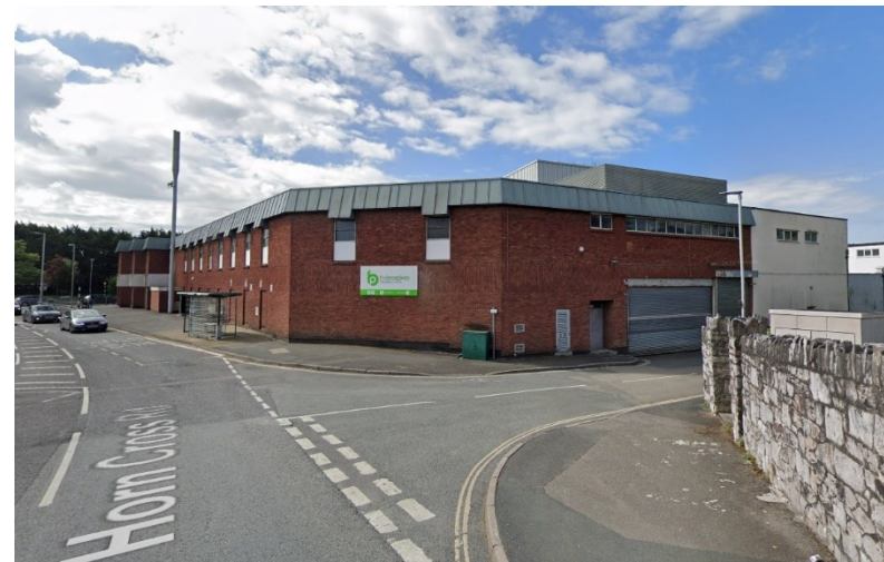
Street views of the existing site
