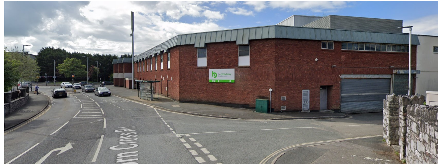
View of site from the north
