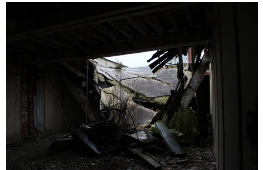
Fig. 3 Photo of collapsed first floor
