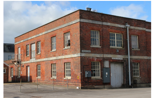
Fig. 1 Photo of the South Elevation
