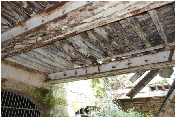
Floor condition in 2021
