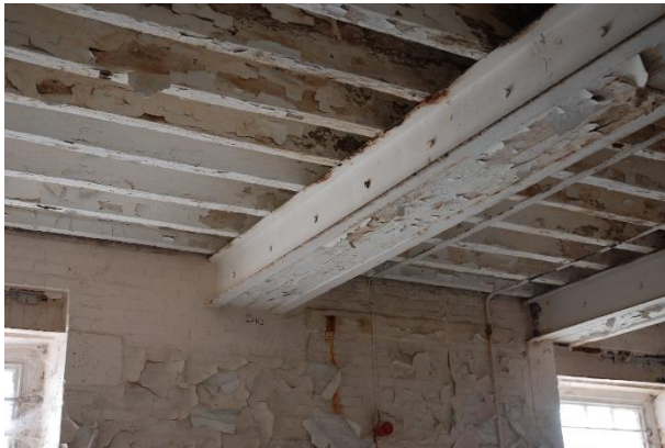
Floor beam in 2021
