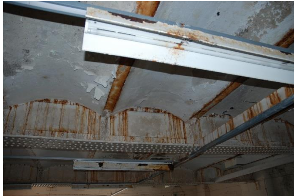
Roof of central section 2021
