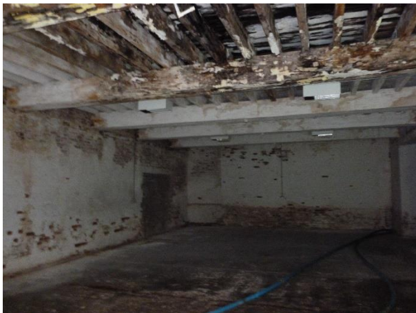
Floor beam condition in 2021
