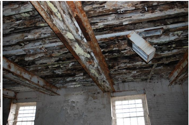
Floor condition in 2023
