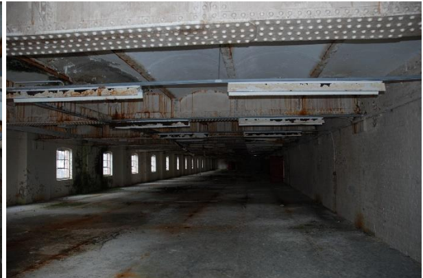
Roof of central section 2023
