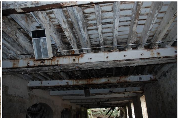
Floor Condition in 2023
