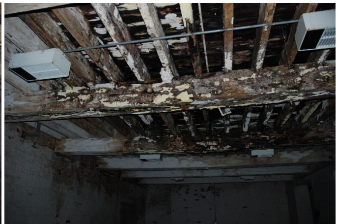
Floor beam condition in 2023
