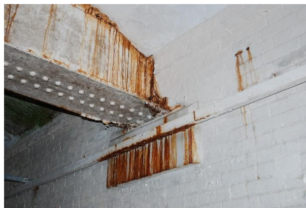
Roof of central section in 2021
