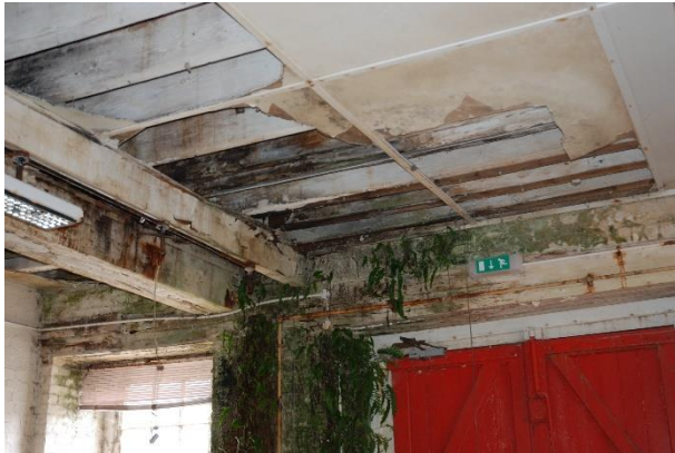
Lintel over door in 2021
