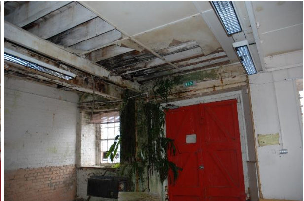
Lintel over door in 2023
