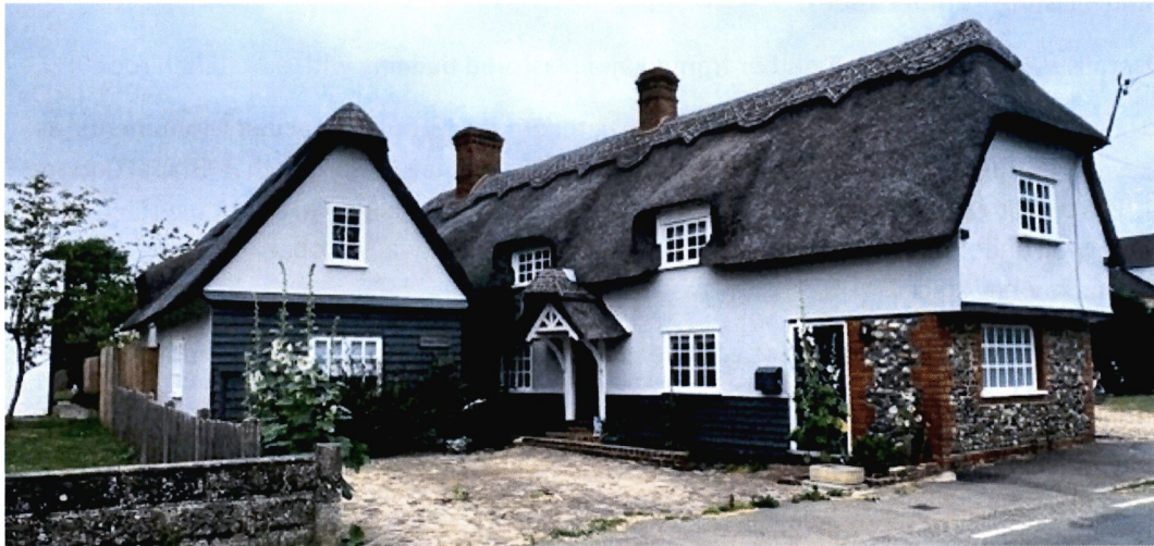
The front of Chapel Cottage and the Outbuilding (June 2023)
