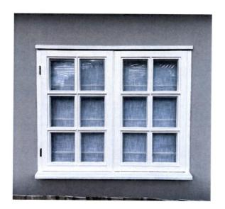
Casement window c 20 years old. Poor thermal retainment.
