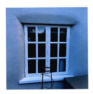
Casement window, c40 years old. Rotten sill and windows. Have been significantly filled. Not watertight or draughproof.
