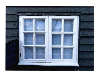
Casement window c 10 years old. Poor thermal retainment.
