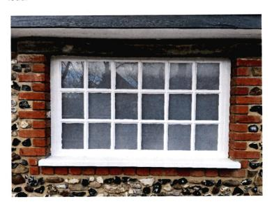
Casement window, c40 years old. Rotten sill and windows. Have been significantly filled. Not watertight or draughproof and acoustically very poor. Road noise is a problem.
