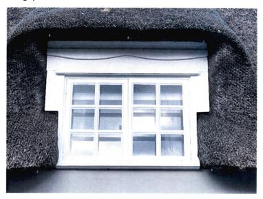
Casement window, c40 years old. Rotten sill and windows. Have been significantly filled. Not watertight, soundproof or draughproof.
