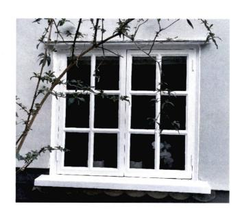
Casement window, c40 years old. Rotten sill and windows. Have been significantly filled. Not watertight or draughproof.
