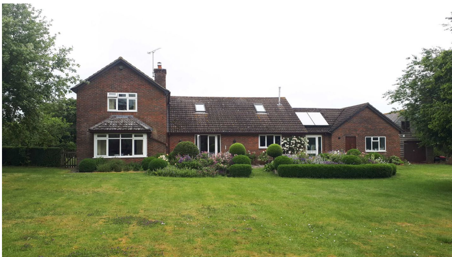
Garden (South) view of the house
