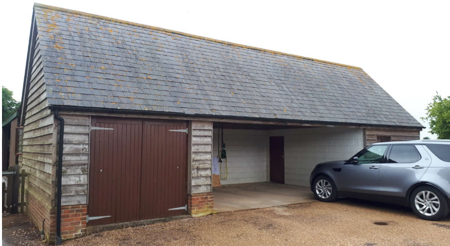
Front (West) elevation of adjacent garage
