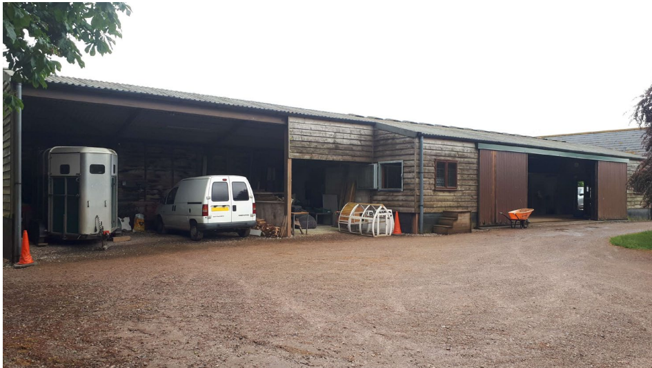
North elevation of the stables behind the garage block
