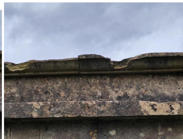
Piecing in to damaged Bath Stone parapet stone
