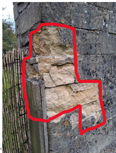
Piecing in to damaged Bath Stone quoins
