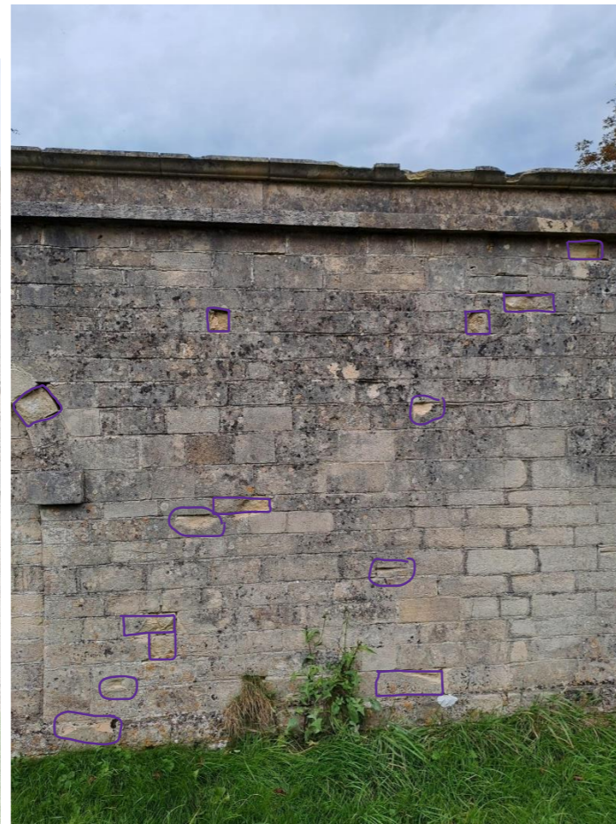
Piecing in to damaged Bath Stone parapet stone
