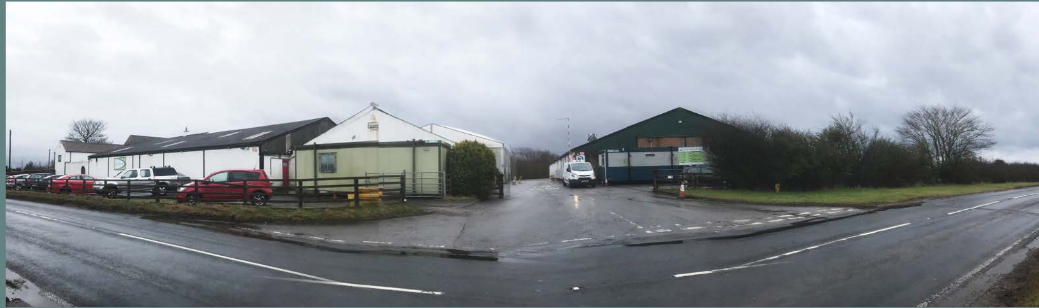
Photo 01 - Existing Access from Thorpe Leazes Lane
