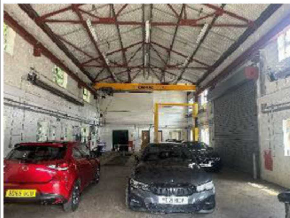
Photo 5: Photograph of corrugated, cement bonded, sheet asbestos containing material and guttering also suspected to contain asbestos
