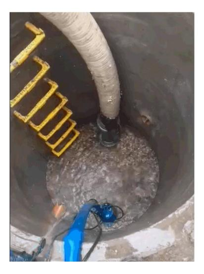
Owing to the health and safety risk associated with deep excavation, confined space, we would not recommend attempts being made to remove the base to lower the unit to the required depth to fit the vortex separator in.
