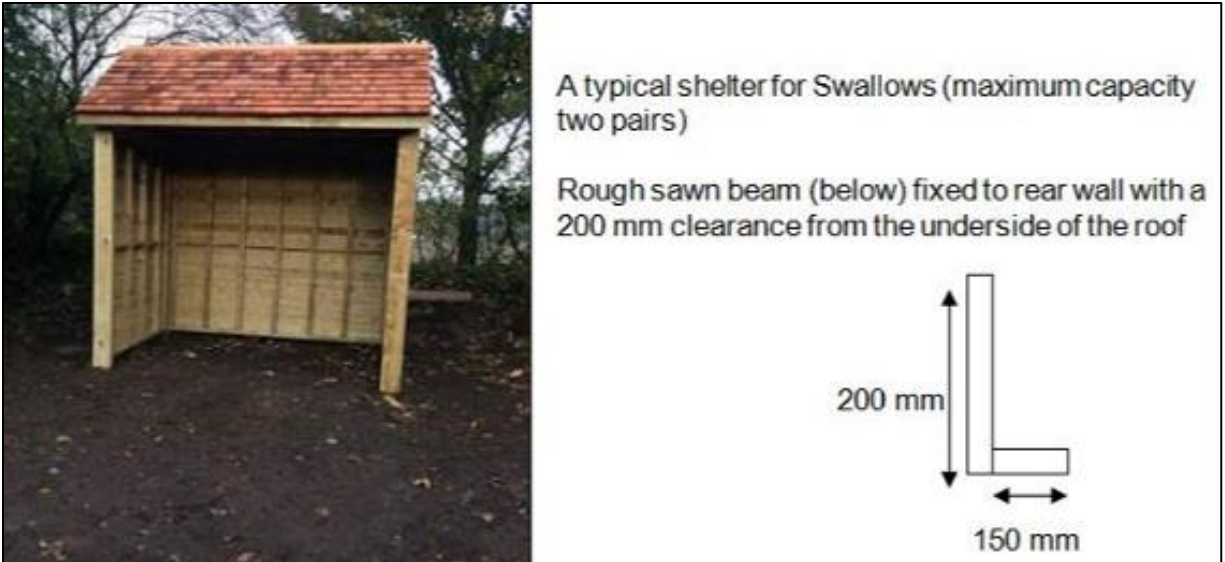
Figure 1 – Example of swallow shelter, a shed with a large opening for access with WoodStone Swallow Nest Bowls may also be used.
