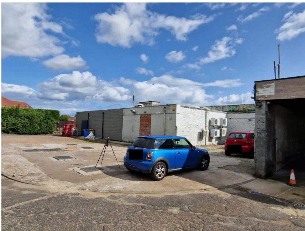
Figure A1.5: View to rear of the Garvock petrol station shop building with view of the eastern boundary open slatted fence on the stone wall (boundary with 88 Halbeath Road) and the large hedge (boundary with 1 Milldean Grove)
