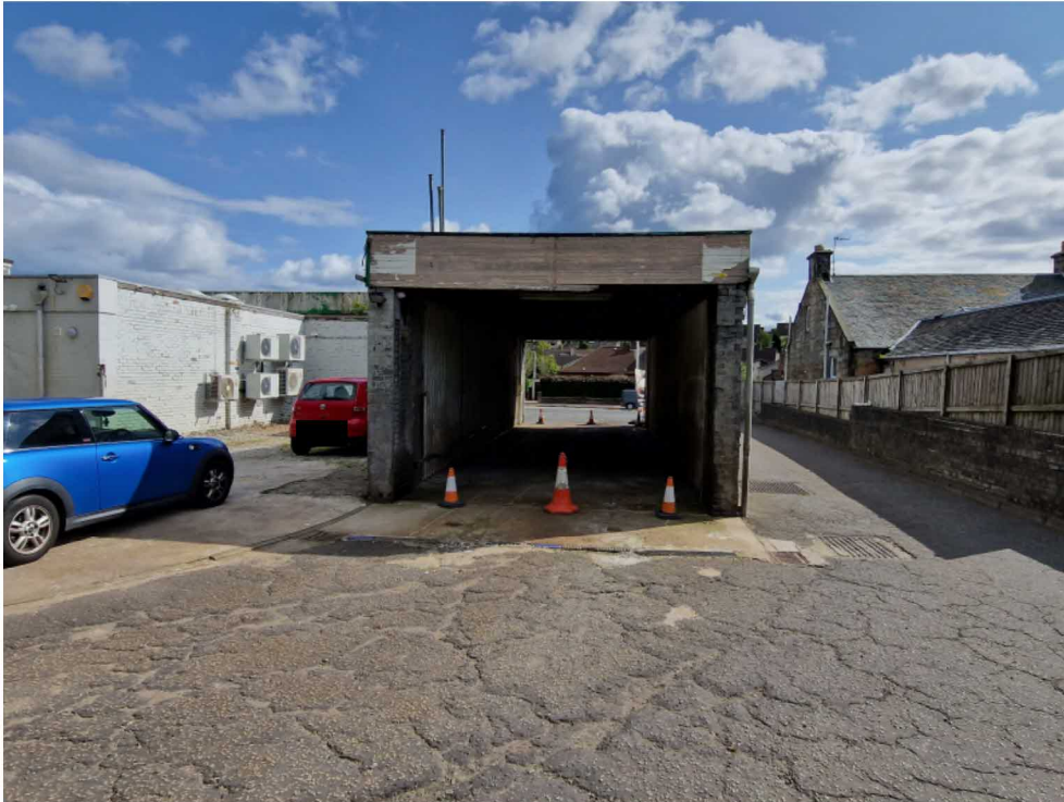
Figure A1.3: View (looking south) of existing carwash portal at Garvock and the wall mounted AC / Refrigeration Units to the left. 82 Halbeath Road and the existing boundary stone wall and fence behind can be seen to the right.
