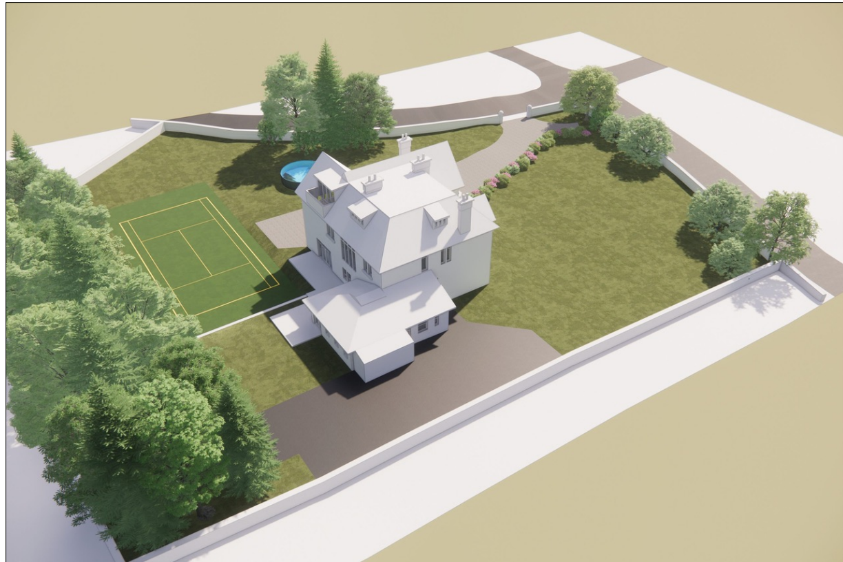
EXISTING north east view
