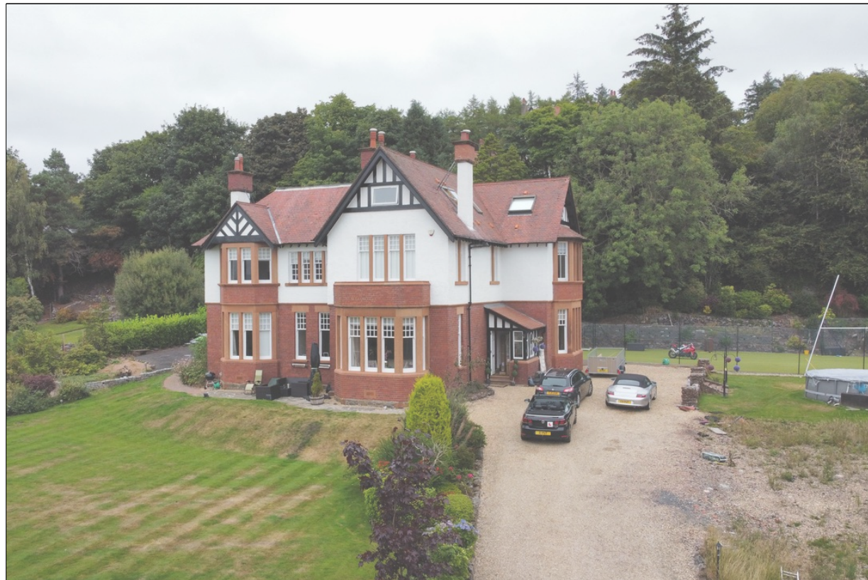
EXISTING south west view
