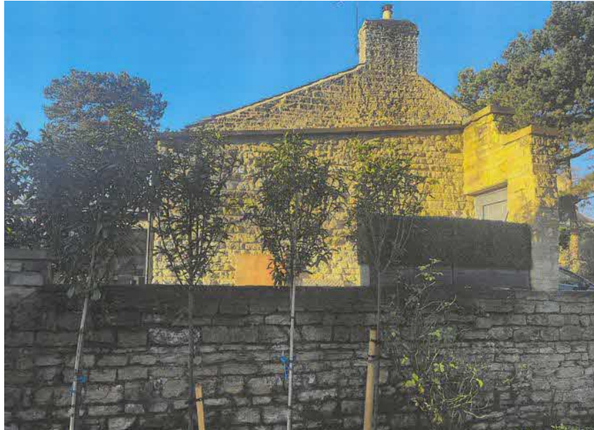
Plate 5 – View of the existing side (northeast) elevation.
