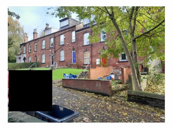
The front garden area of the property has been significantly excavated with large brick retaining walls to either side. These engineering works are unauthorised, and will be replaced/removed..
