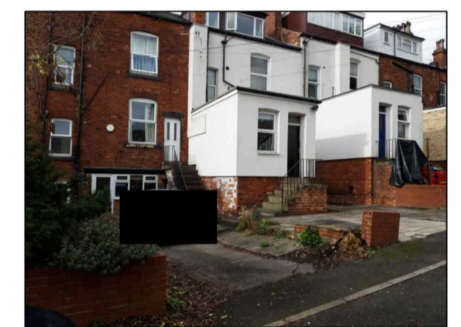
Photo of rear elevation
