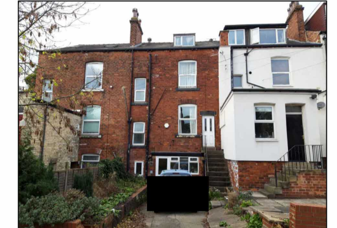
Photo of rear elevation
