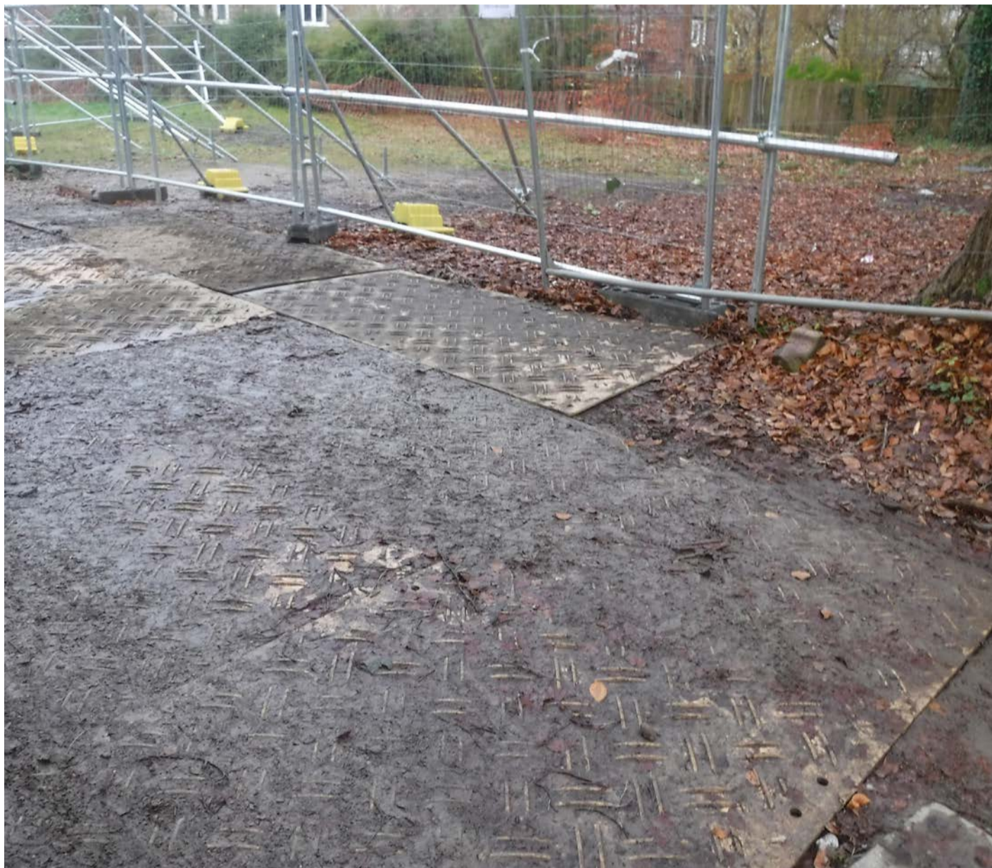
Ground Protection Guards in Tree Protection Area
