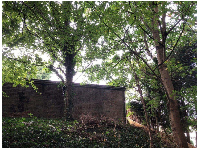
Photo 3: T7 & T8 reduction away from building
