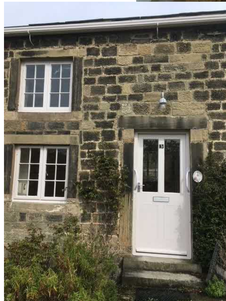
Photograph from 2019 illustrating the original Steps to the main entrance and varied casement types to the ground and first floor windows.
