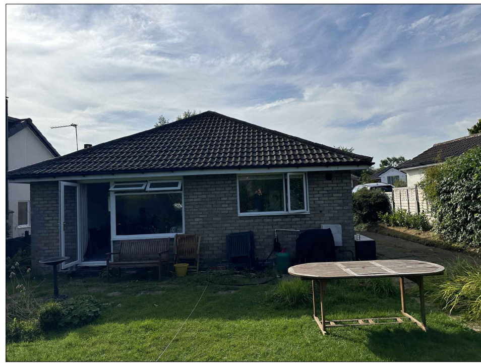
Photo 1 Rear Elevation As Existing
