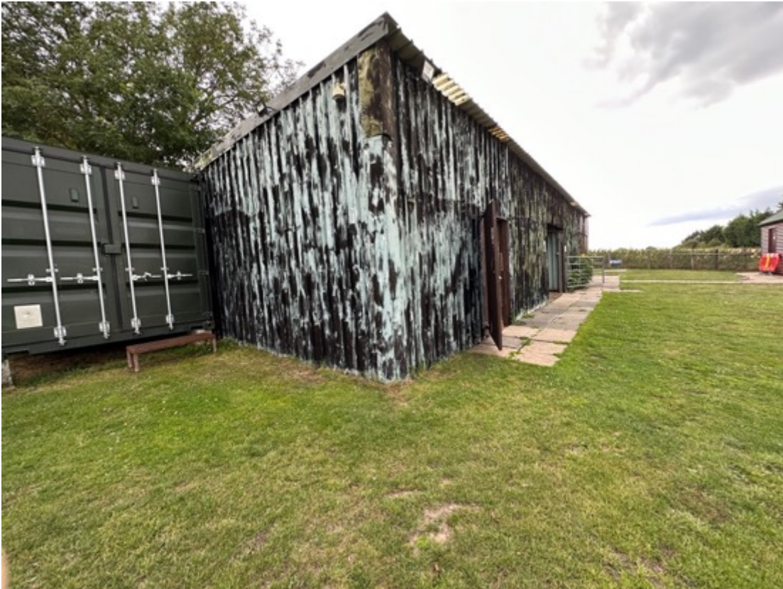
Photograph 3: Side (east) of the building, looking south-west
