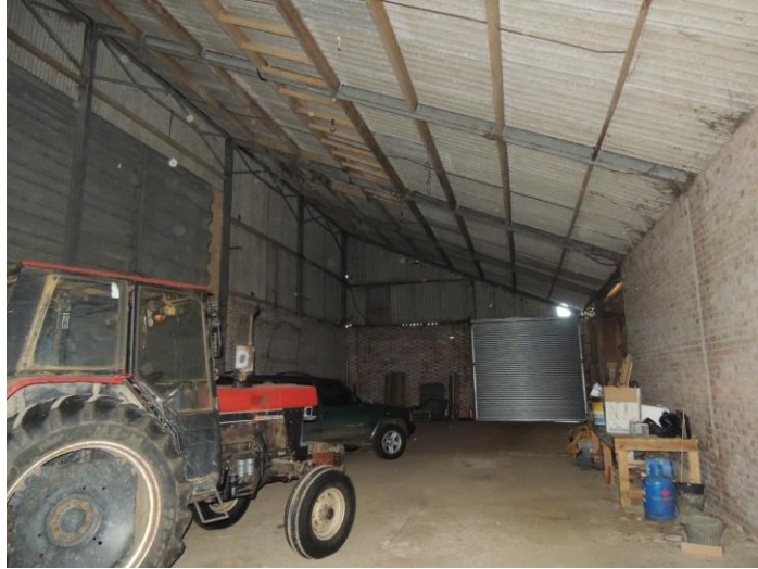
Photo 8: Looking S-N in the building
