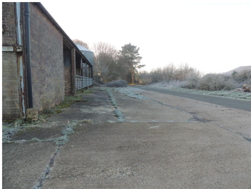
Photo 14: Showing road and extent of concrete hardstanding to west
