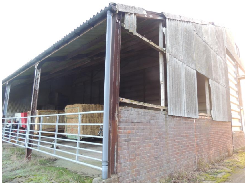
Photo 4: The south-west corner
