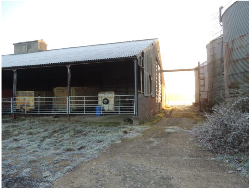
Photo 18: Showing proximity of silos to southern end of barn
