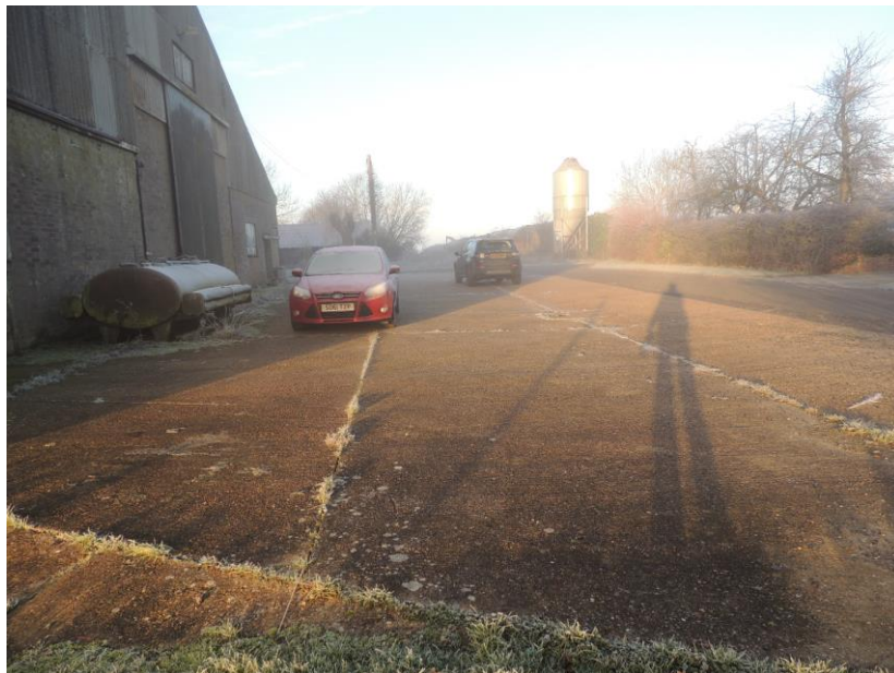
Photo 12: Showing road and extent of concrete hardstanding to north
