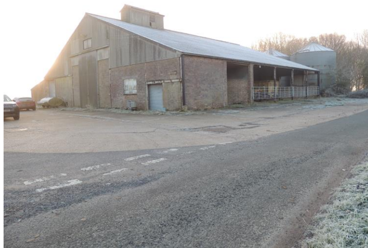
Photo 17: View from north-west showing extent of hardstanding
