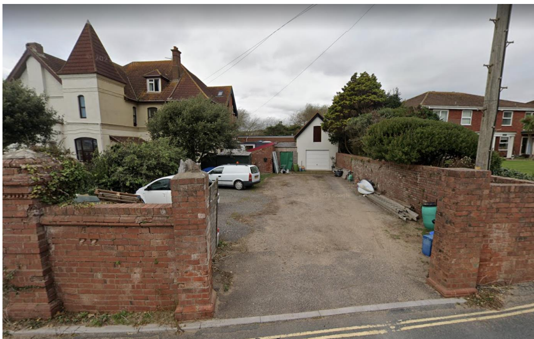
View into the proposed site from Maer Lane, white outbuilding to right hand side is to be demolished
