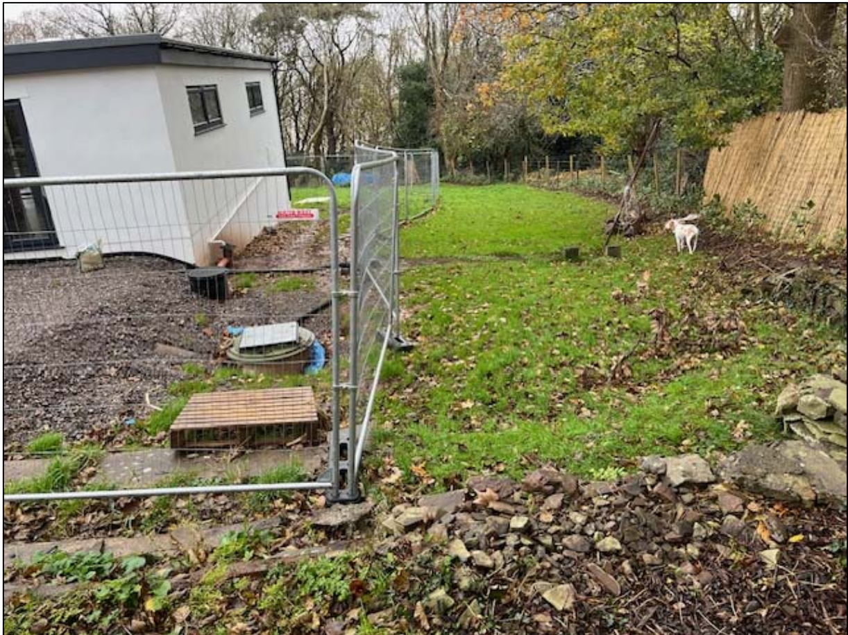
Figure 2: The tree protection fencing has been in place throughout the construction works.
