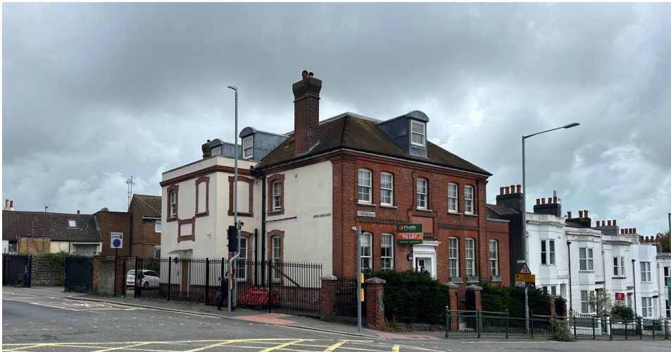
Railings as reinstated.
