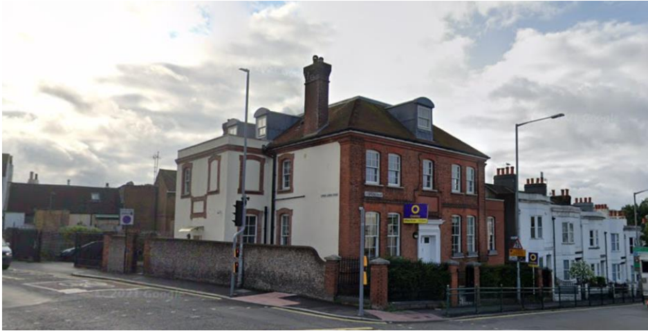
Wall prior to damage by car:
