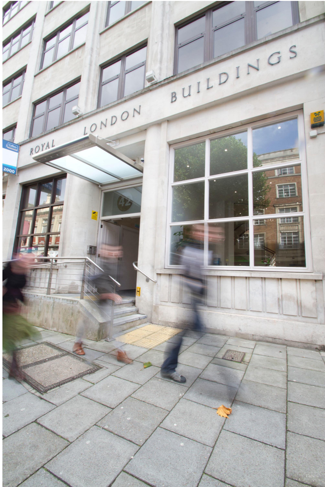
▲ Existing entrance to the Royal London Buildings
