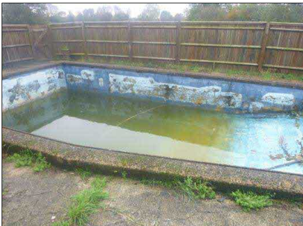
Photograph 13 Showing the swimming pool
