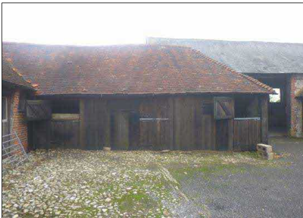
Photograph 7 Showing Building D
