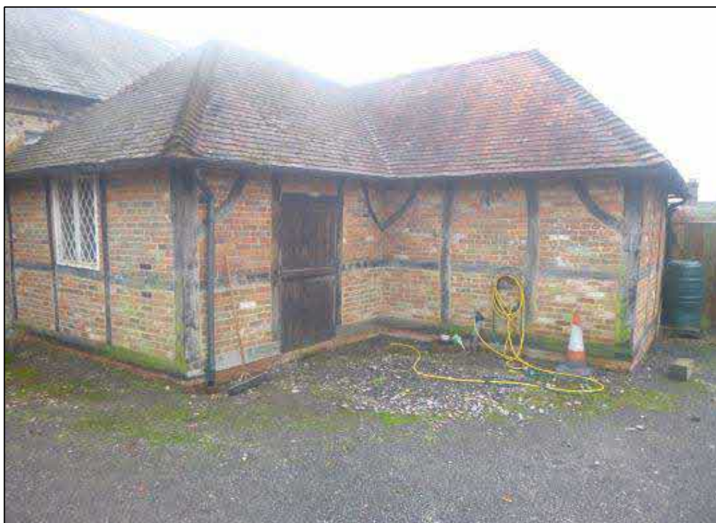
Photograph 11 Showing Building F
