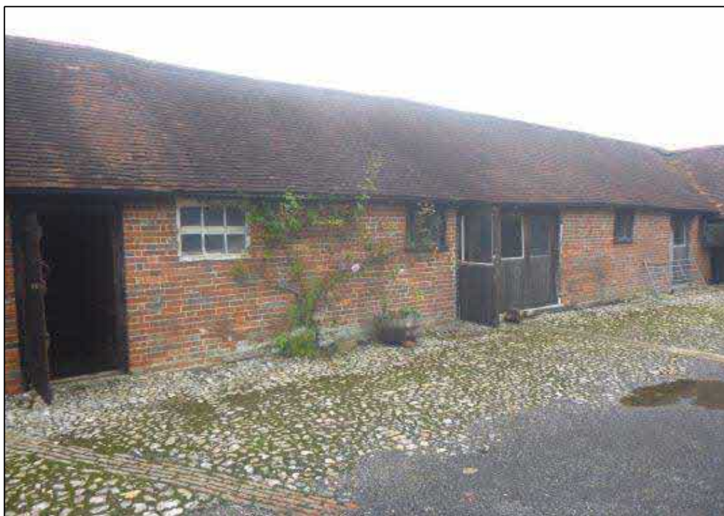
Photograph 5 Showing Building C
