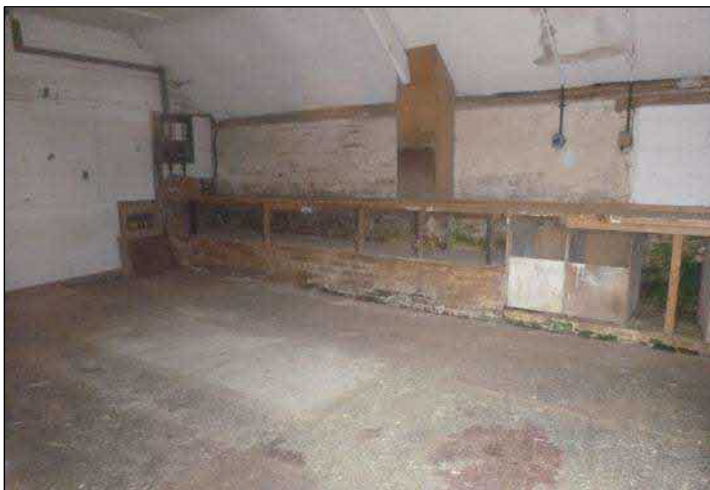
Photograph 6 Showing inside Building C
