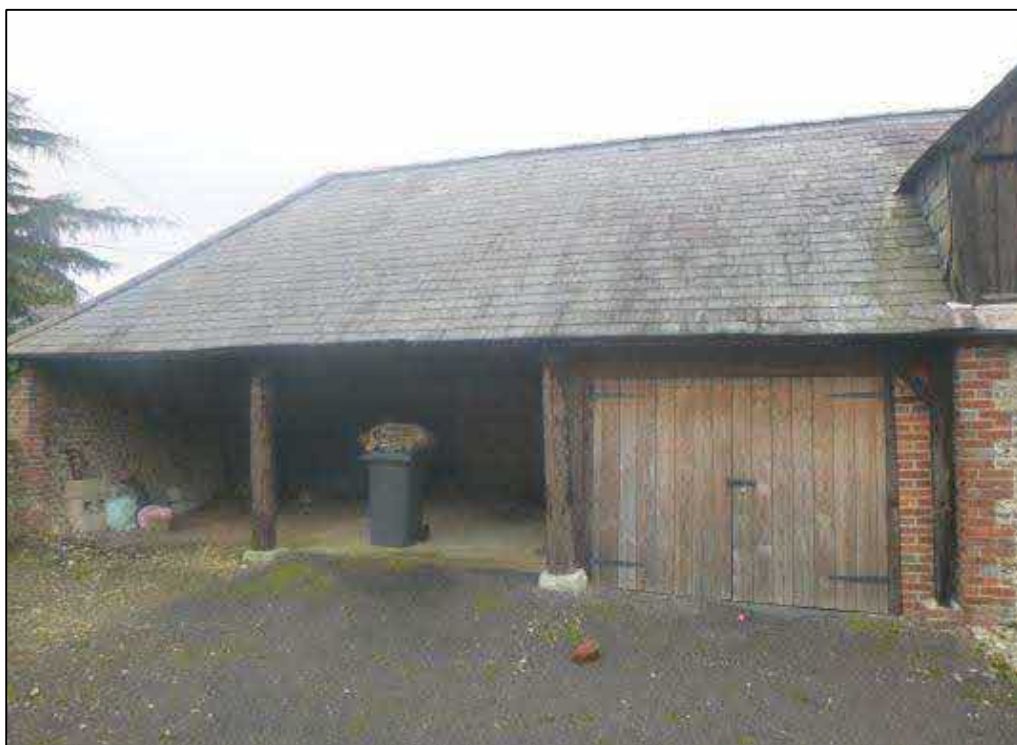
Photograph 2 Showing Building A
