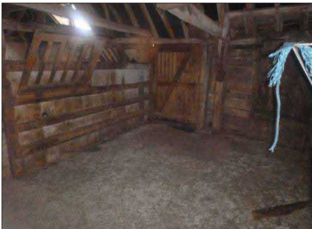
Photograph 8 Showing inside Building D
