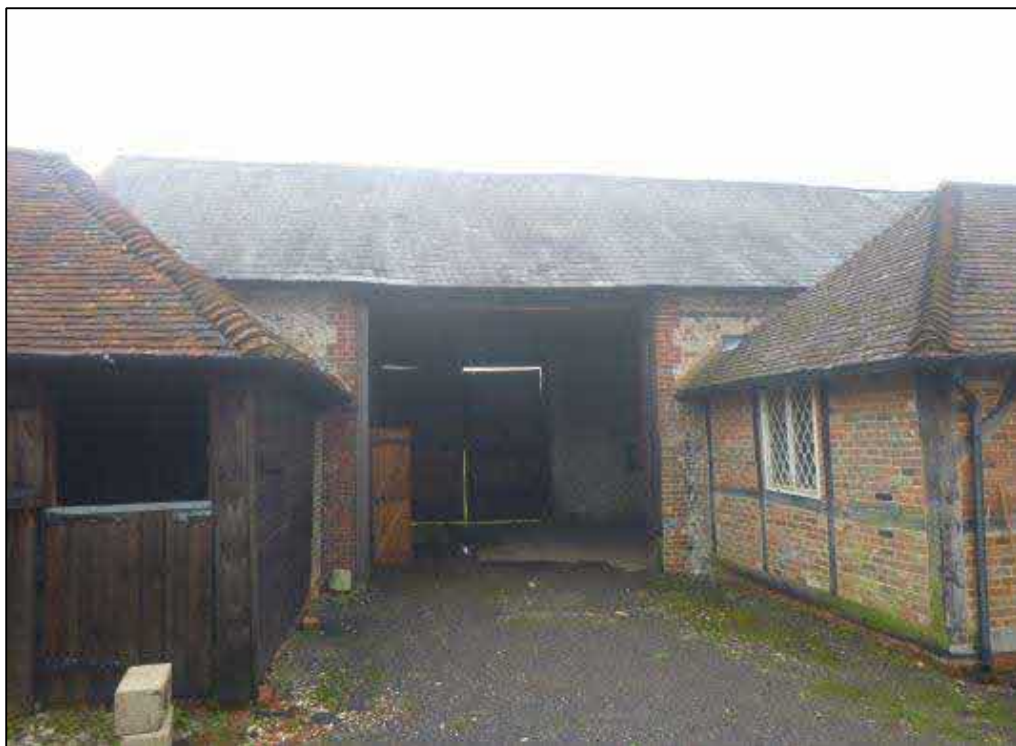
Photograph 9 Showing Building E
