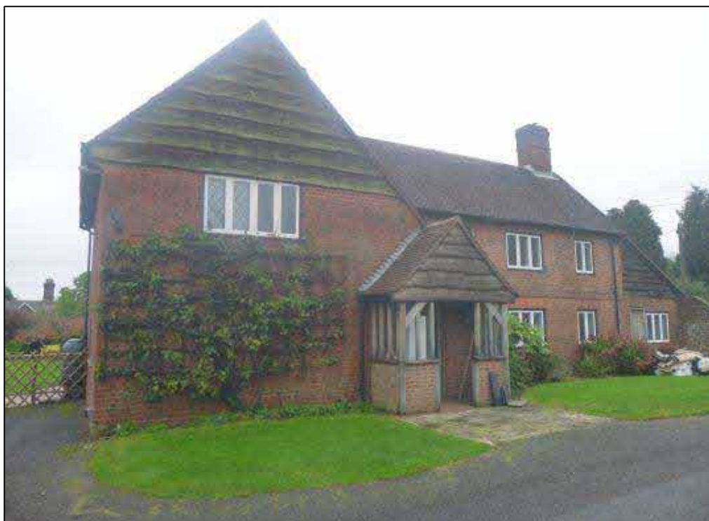
Photograph 12 Showing Building G
