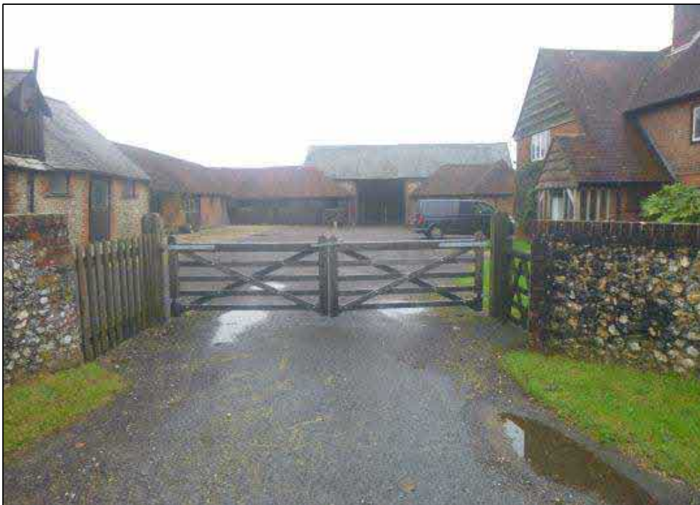
Photograph 1 Showing the entrance onto the site
