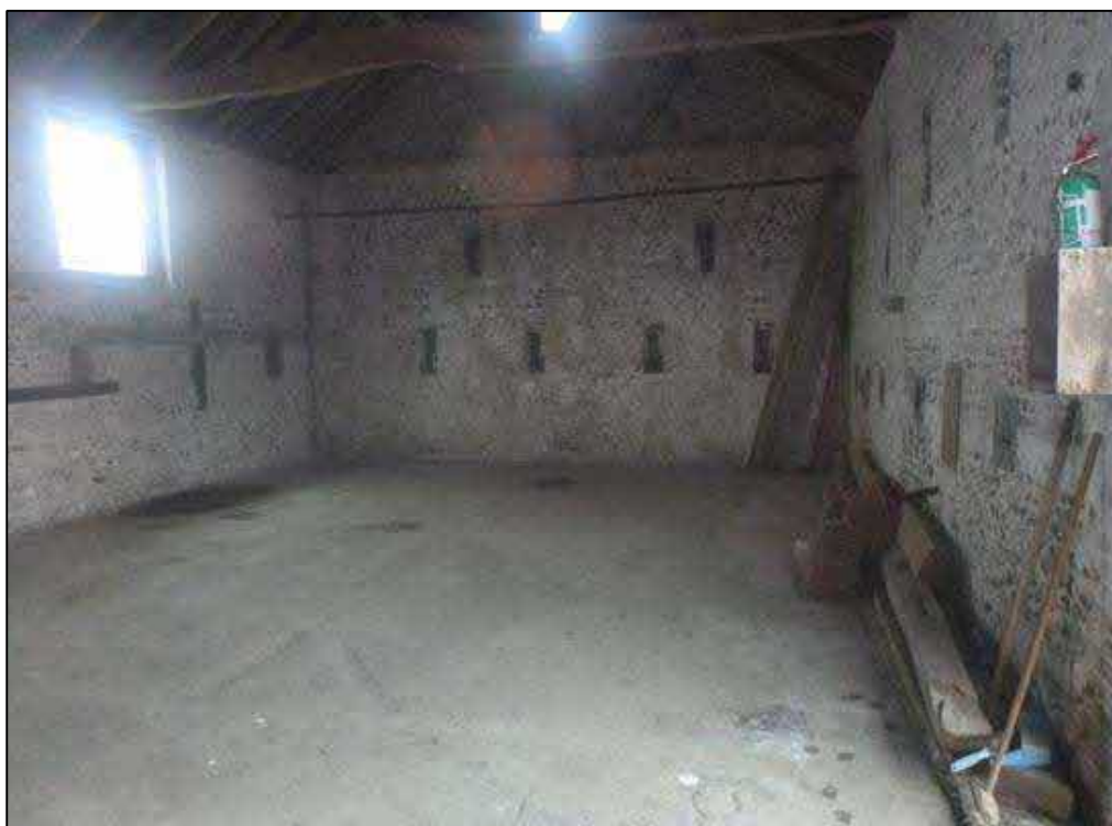
Photograph 10 Showing inside Building E
