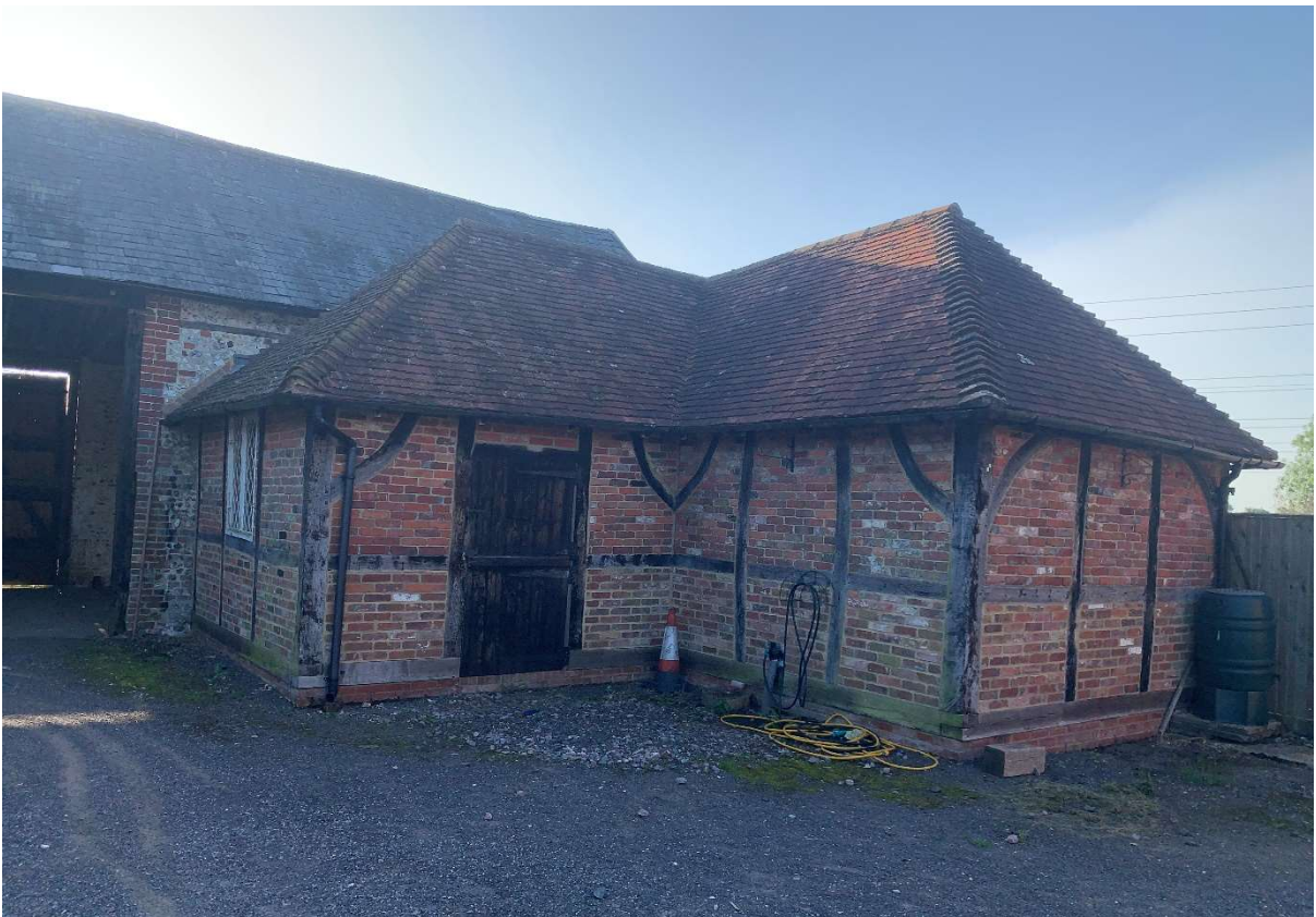
Figure 4: Existing timber framing with brickwork infill panels
