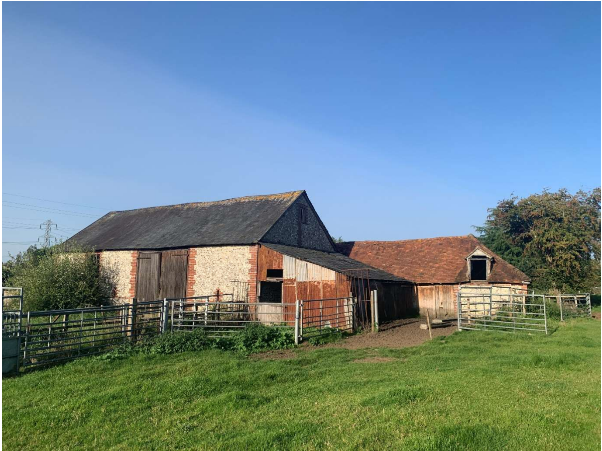
Figure 5: Existing slate and clay roofs, timber dormer and corrugated sheeting
