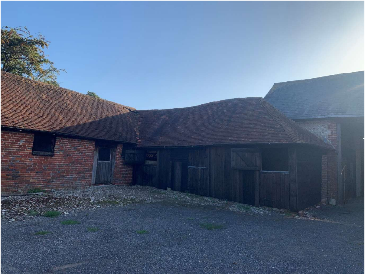
Figure 3: Existing timber cladding to stables
