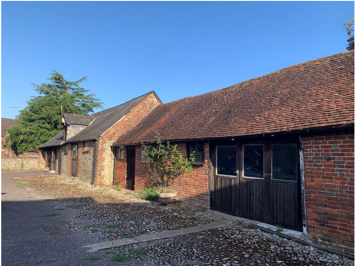
Figure 2: Existing clay tiles, brickwork, and timber fenestration
