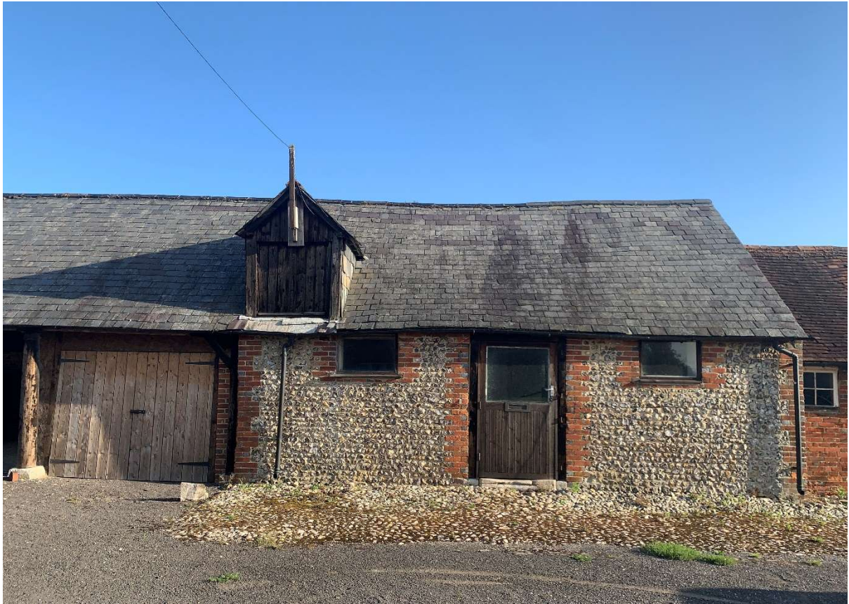
Figure 1: Existing slate tiles, flintwork, cobbles and gravel
