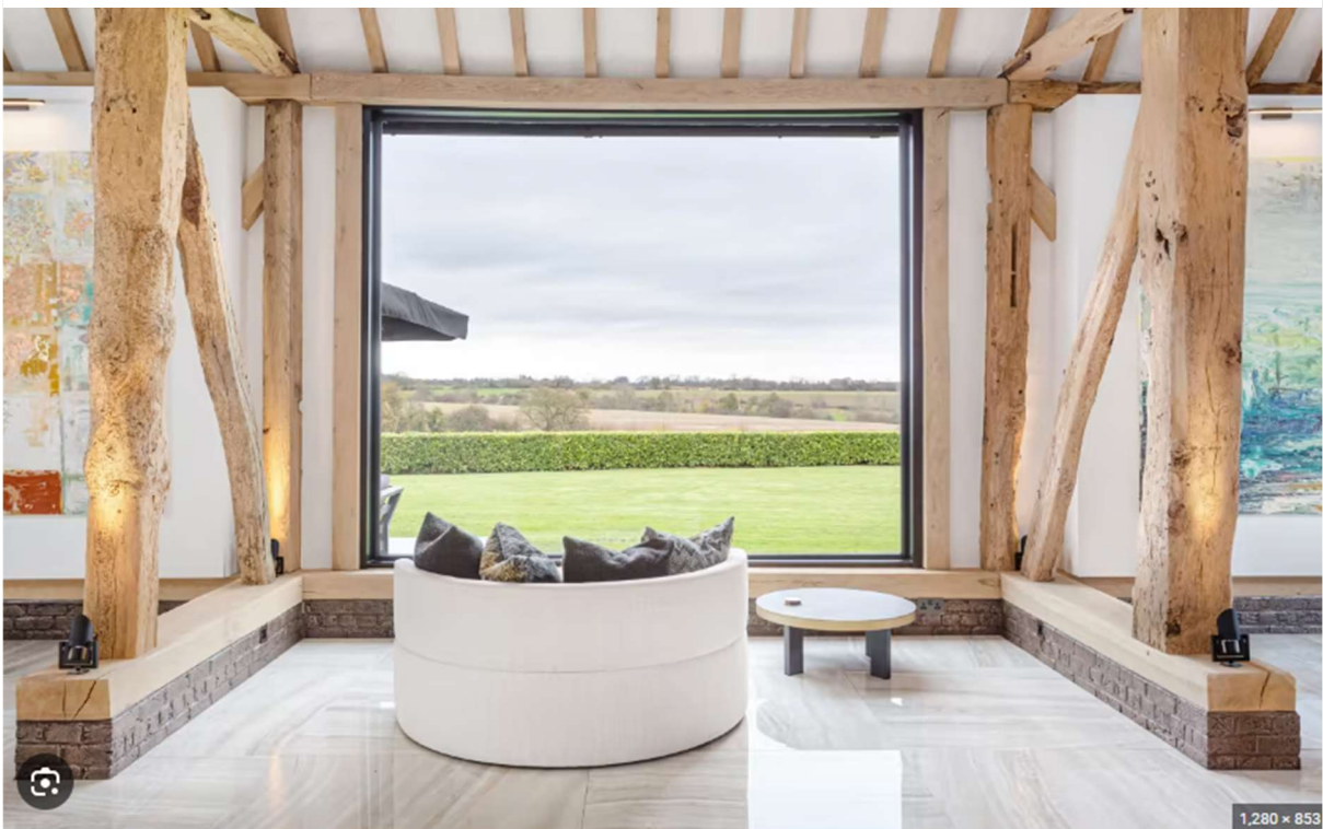
Figure 11: Proposed slim frame glazing with timber framing
