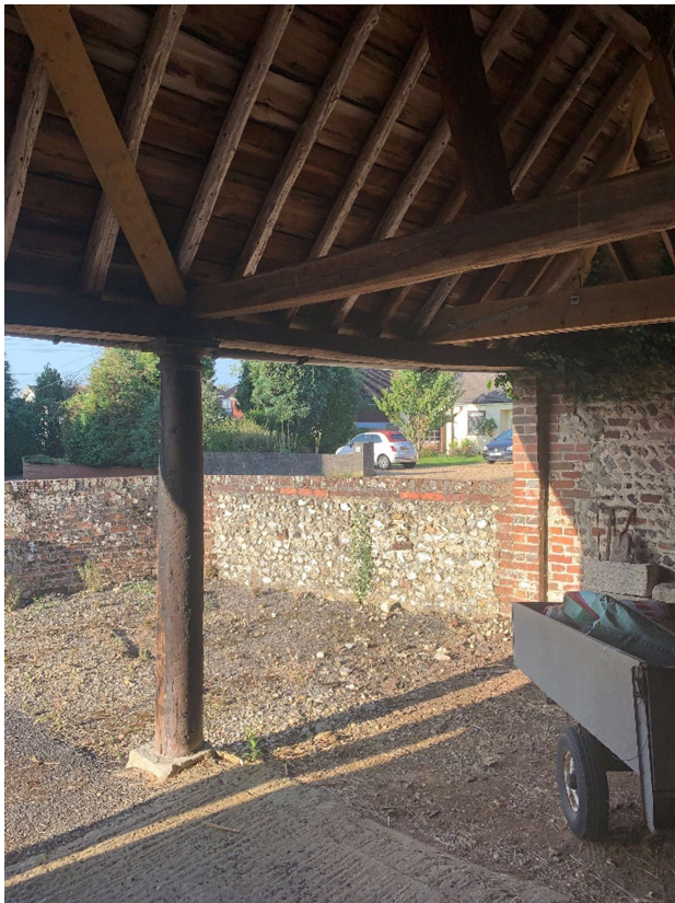
Figure 6: Existing front boundary wall (flint and brick)
