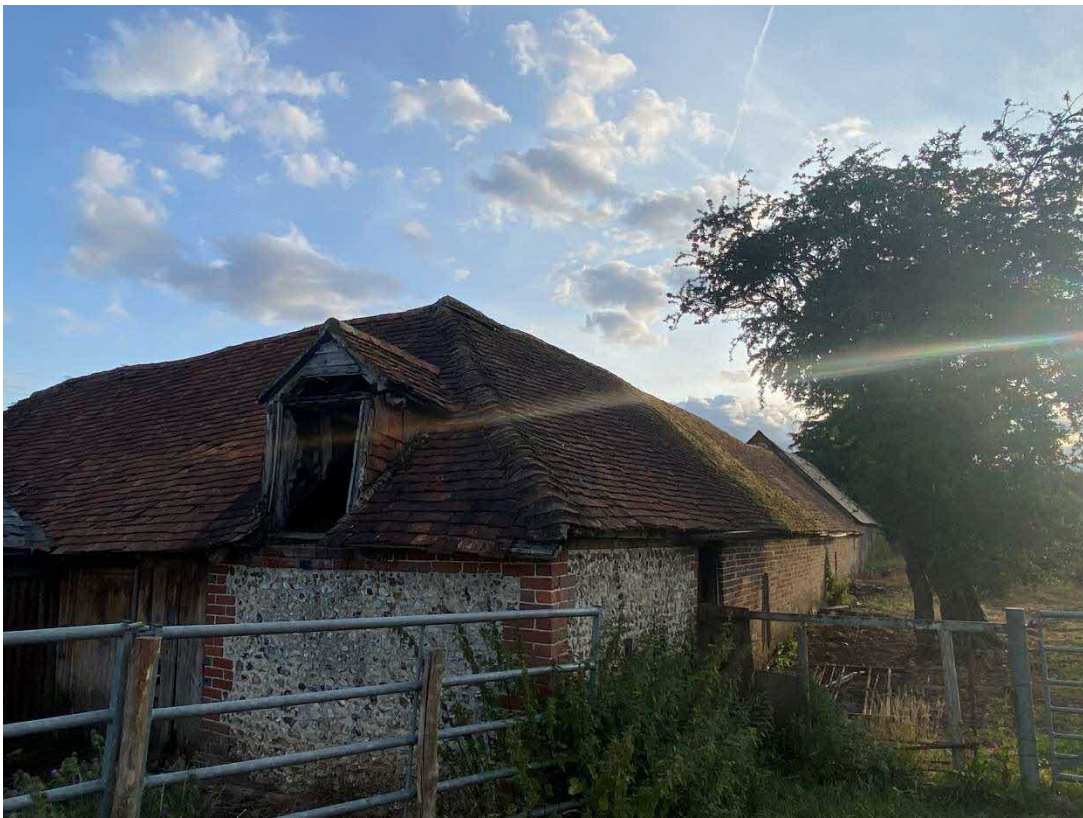
Figure 8. Middle Building Eastern and northern elevations looking west.
