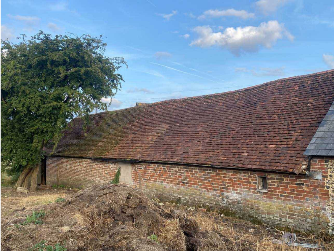
Figure 7. Northern elevation of Middle building looking southeast.
