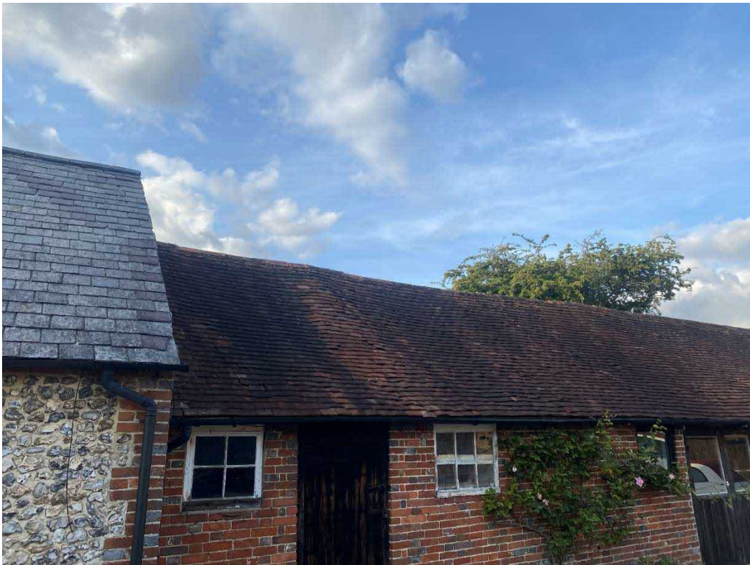
Figure 5. Southern elevations of western third of Middle buildings looking northeast.
