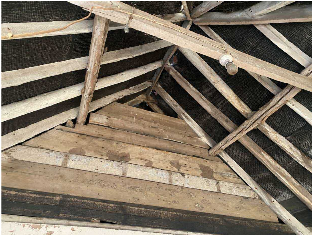
Figure 13. Interior of open (south) section of south building looking west.
