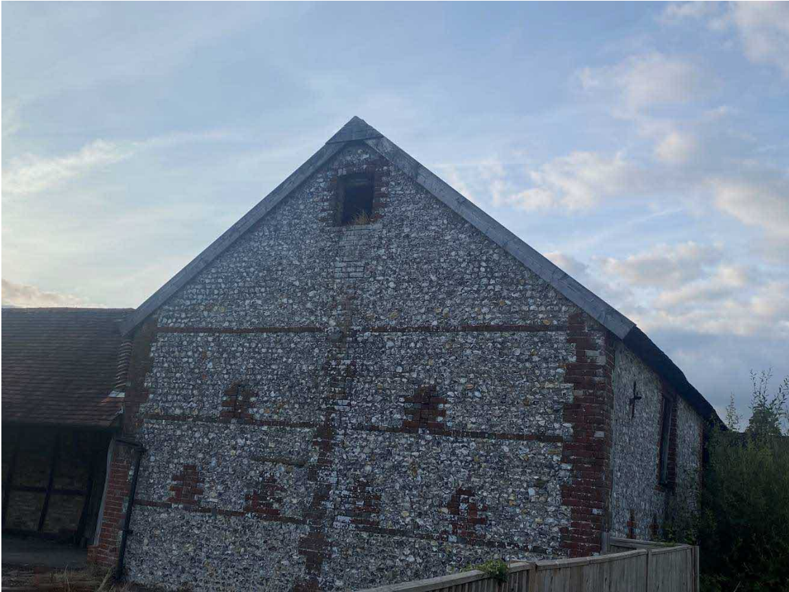
Figure 8. Southern and eastern elevations of east barn looking north.
