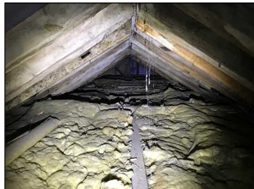
Figure 10 – internal view of the westernmost void
