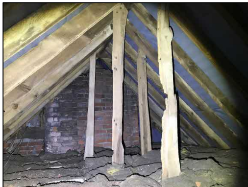
Figure 9 – internal view of the easternmost void
