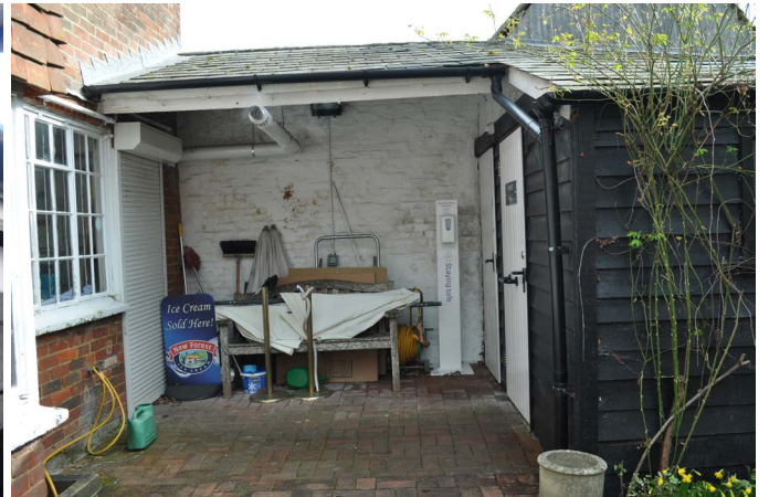
Existing open recessed area of lean-to
