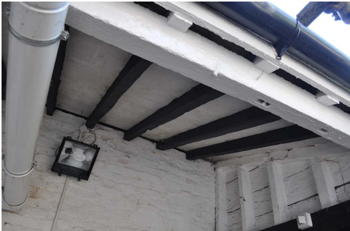
Existing historic roof structure
