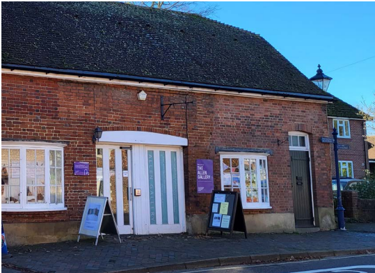
Existing carriageway entrance to gallery
