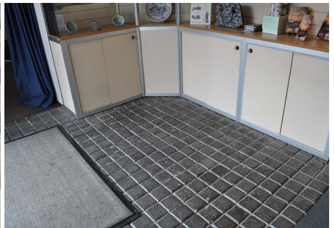
Existing stable brick floor finish to lobby to be retained
