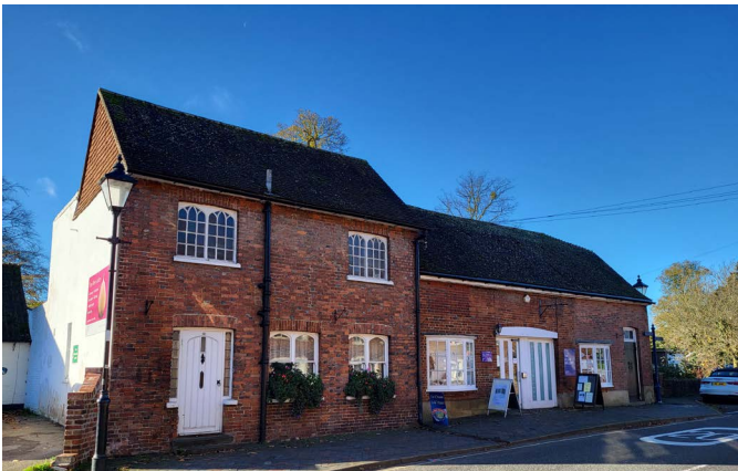
Principal elevation on Church Street
