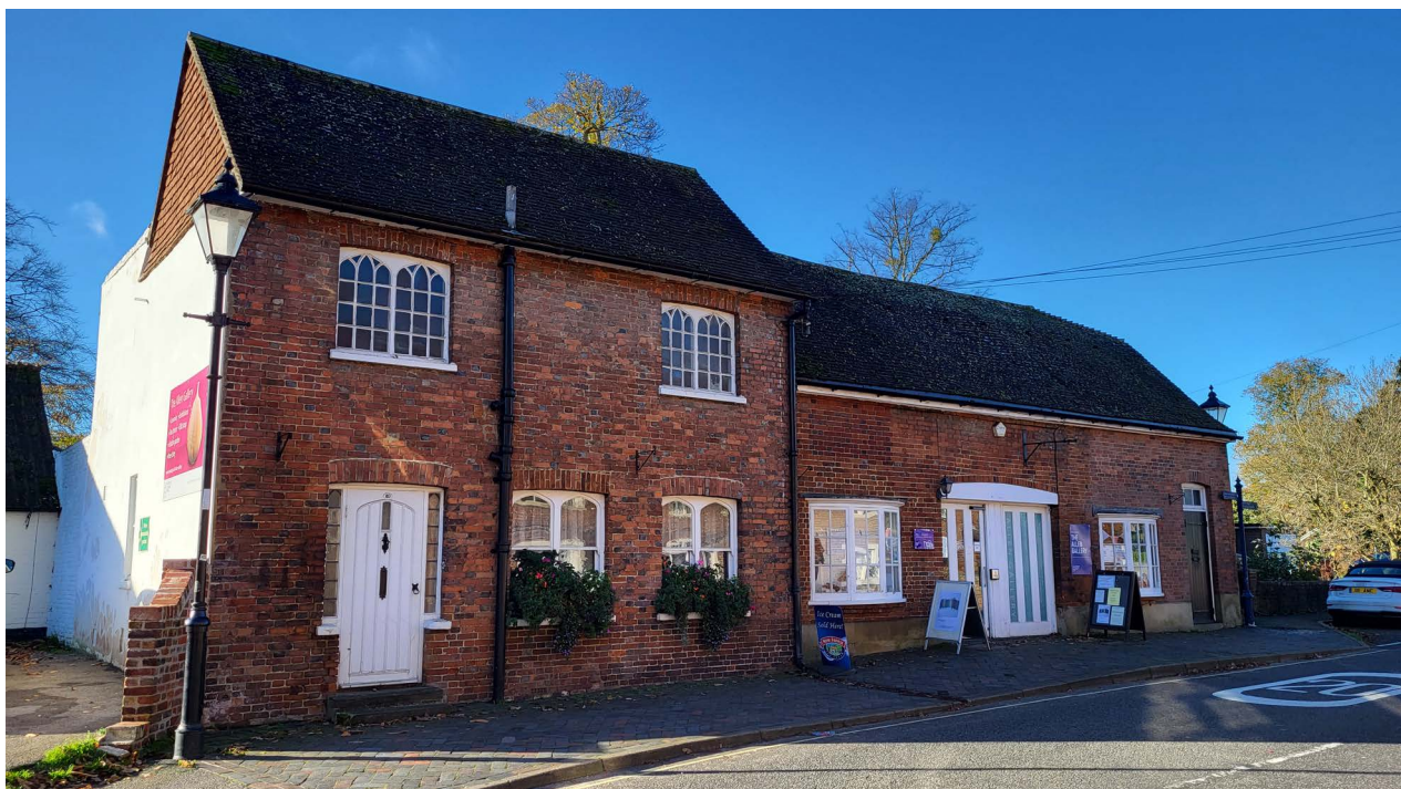
Street Elevation of the No. 10 & 10a Church Street
