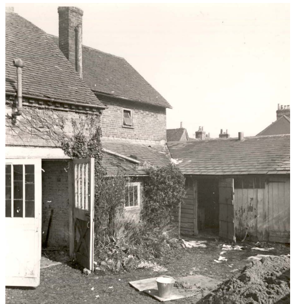
1952 Photo of rear of No. 10 and 10a
