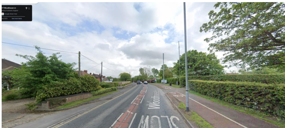
Figure 4 - Roadside View Looking East (Google Maps)
