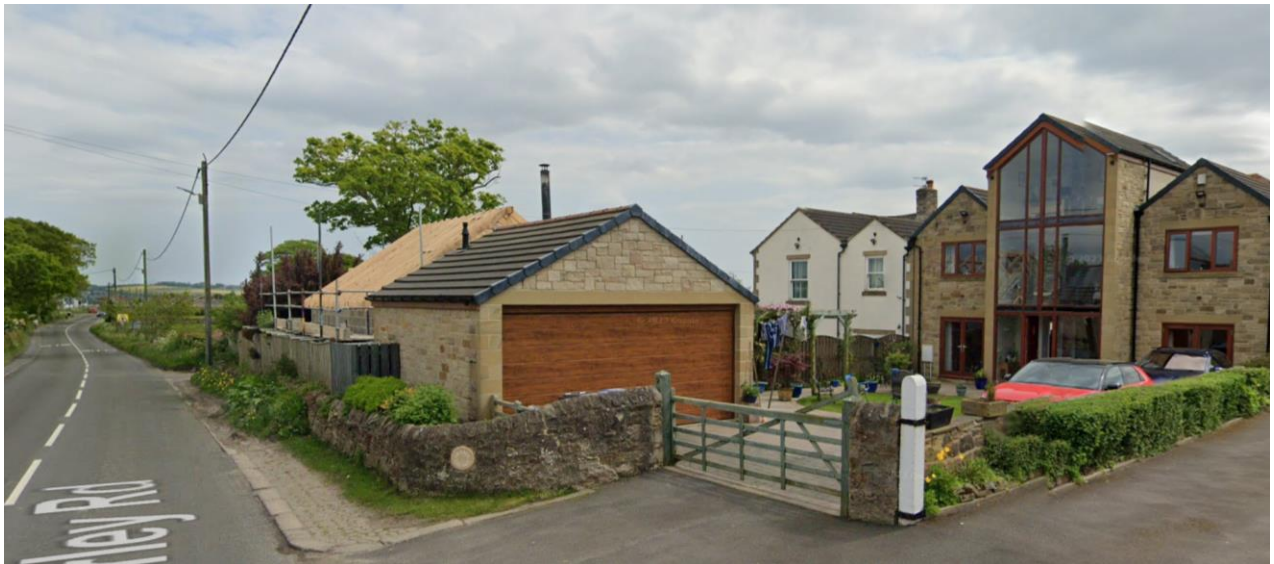
Figure 5 - Garages at Etherley Grange
