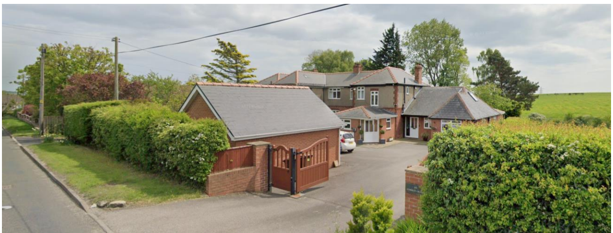
Figure 6 - Garage at Etherley Grange
