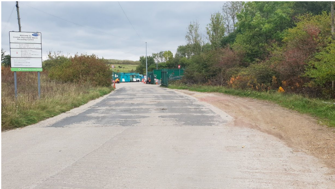
Figure 2.4 – Photograph of the entrance of Coxhoe Household Waste Recycling Centre and access route to the proposed leachate treatment facility
