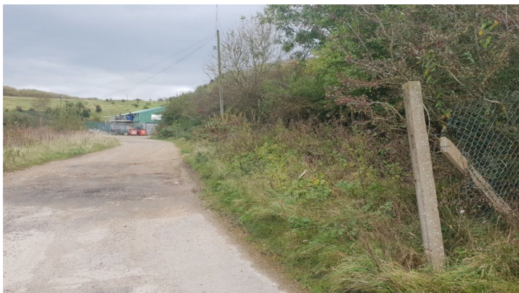
Figure 2.2 – Photograph of the application site looking east, with the access track to the north and the gas utilisation plant in the near distance
