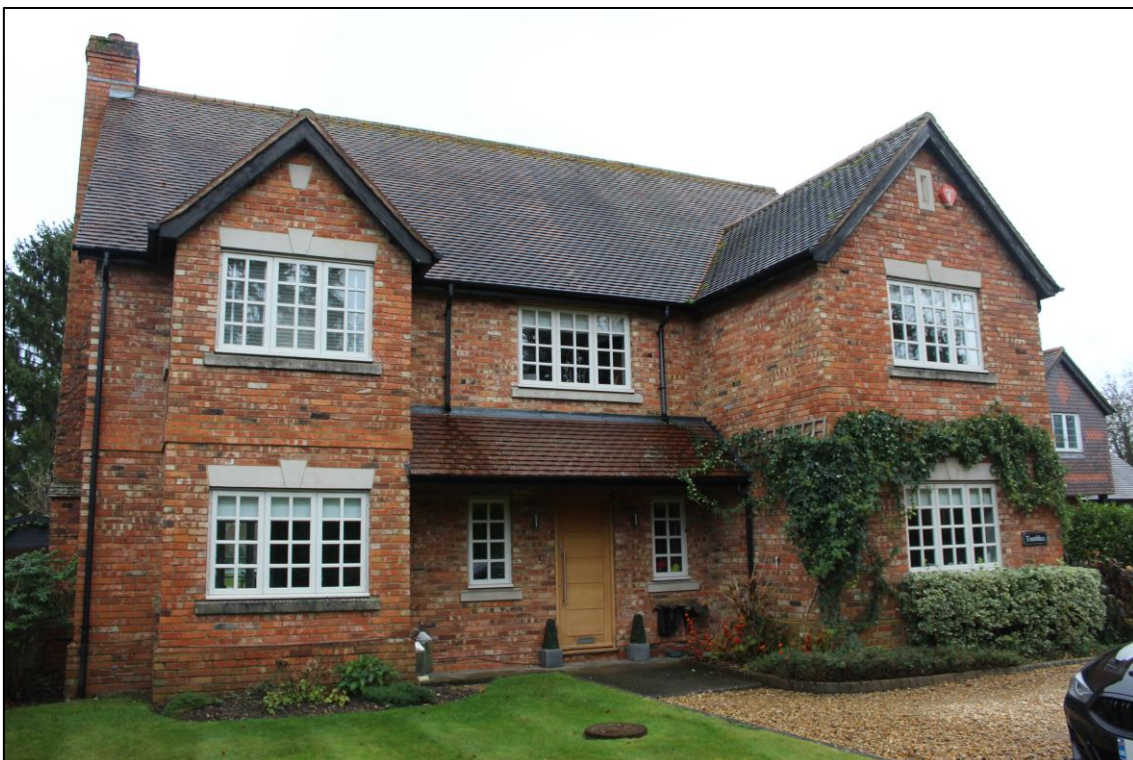
Photograph 1- Front elevation as viewed from the driveway
