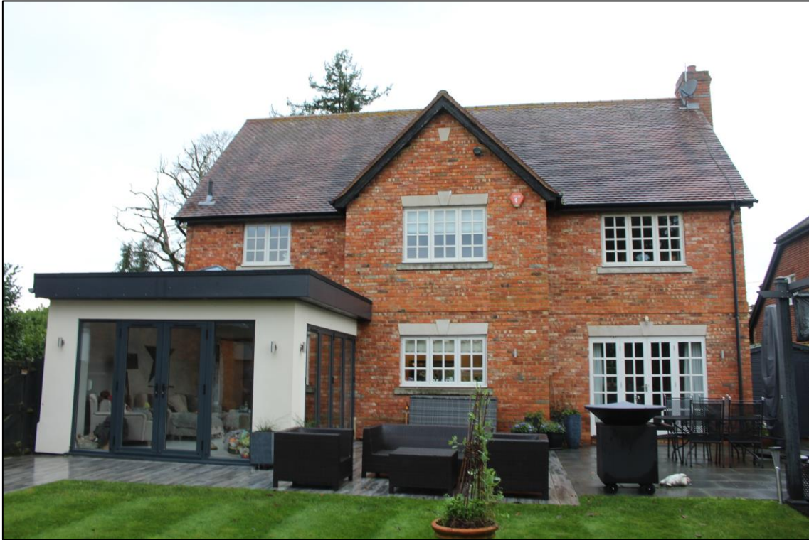
Photograph 2- Rear elevation showing single-storey rear extension as viewed from the garden
