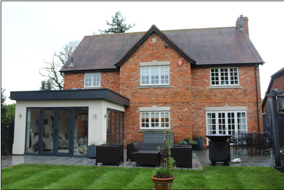
Photograph 2 – Rear elevation as viewed from the garden
