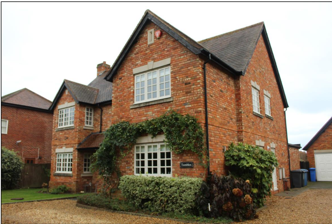
Photograph 1- Front elevation as viewed from the driveway
