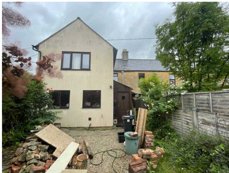
Figure 2- Existing South Elevation
