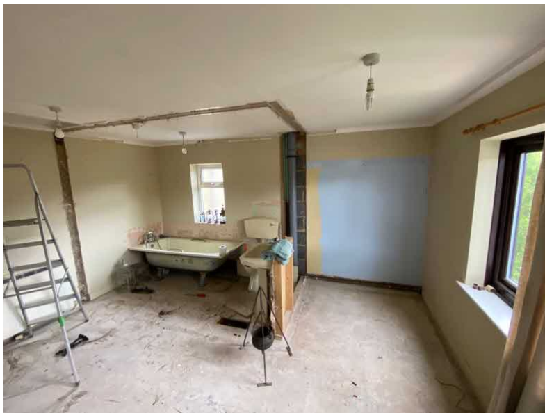
Figure 7 – Existing bathroom in bedroom 3
