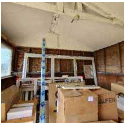
Photograph 5: Internal view of stable block.
