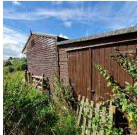
Photograph 4: Eastern elevation of the stable block.
