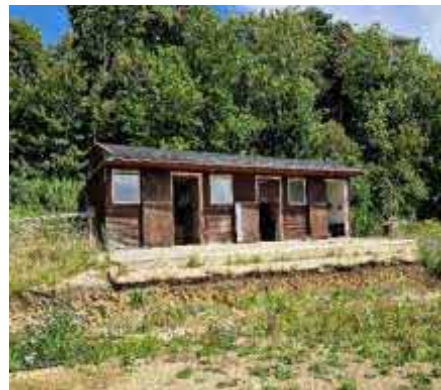
Photograph 6: Southern elevation of stable block and modified habitats surrounding.
