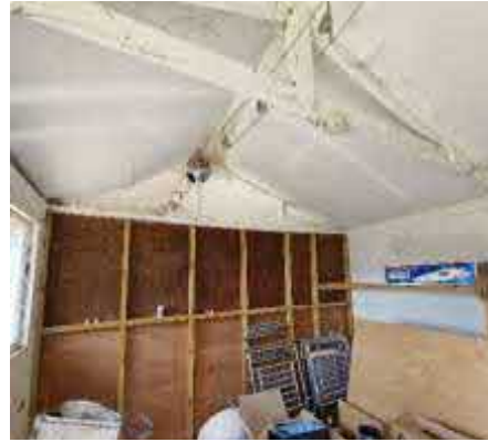
Photograph 2: Internal view of the stable block.
