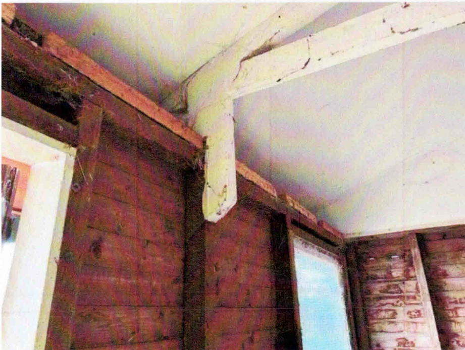
PLATE D -- TRUSS SUPPORT AT FRONT WALL
