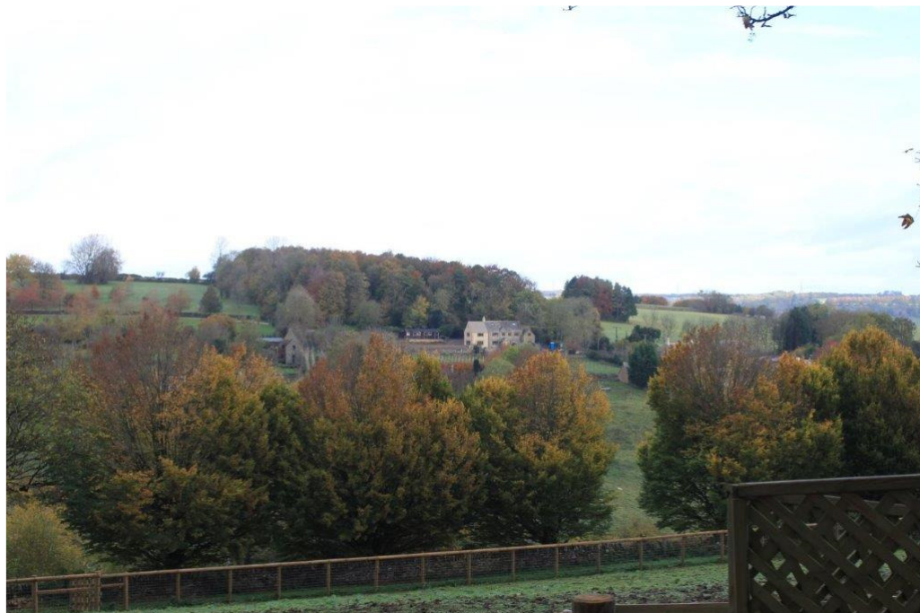
Whilst visible in longer distance views from the lane adjoining No.1 The Hemplands, the stables building is not prominent and is clearly set within the context of the extended dwelling.
